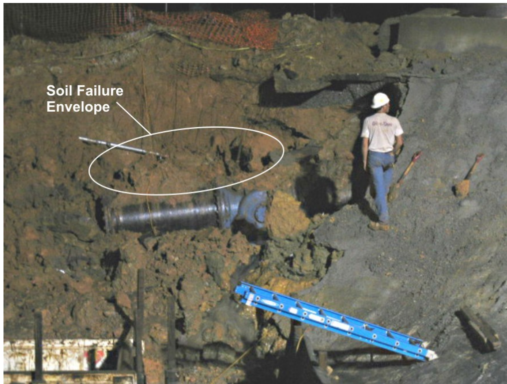
Figure 3-6. Soil Failure Surface, Approximately 10 feet into Slope, June 2006
