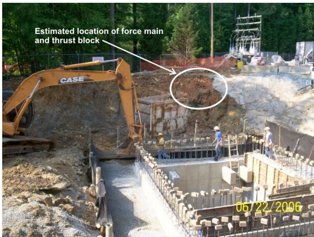
Figure 3-5. Excavation for Placements of Concrete, June 22, 2006
