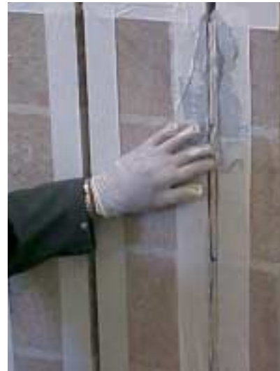
(b) Encapsulation of FRP Bar
