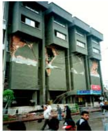
(b) Failure due to In-Plane Loads
