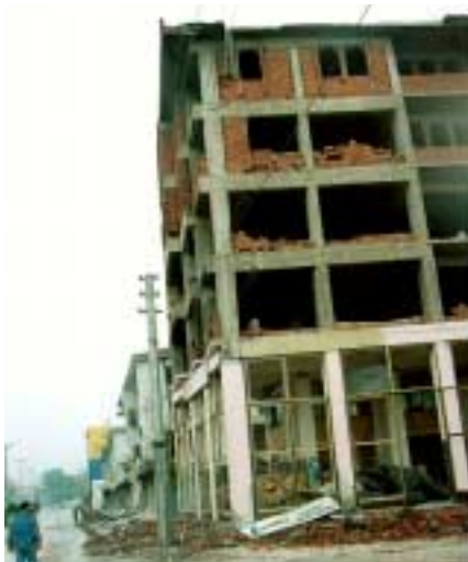
(a) Failure due to Out-of-Plane Loads
