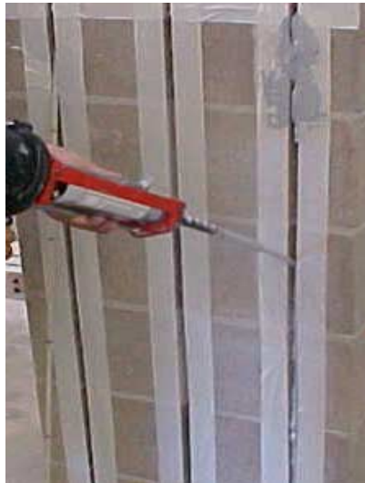
(a) Application of Embedding Paste
