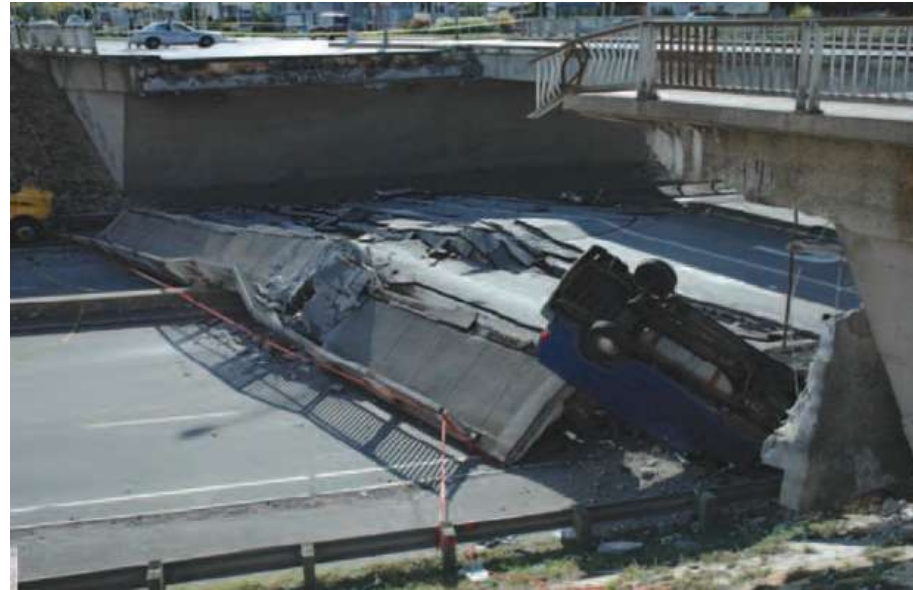
Shear failure of the de la Concorde bridge, Laval
