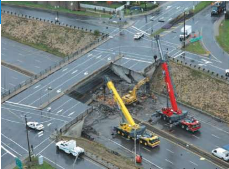
Shear failure of the de la Concorde bridge, Laval
