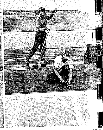
No roofing delays. Nail or mop 43 lb base sheet.
