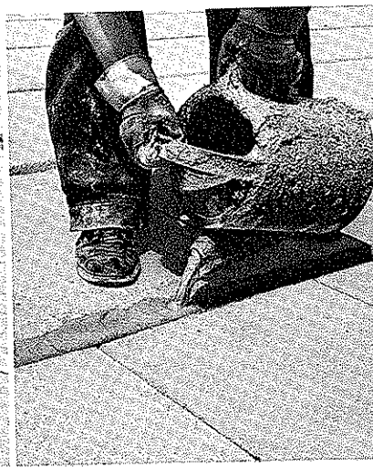
Pre-mixed grout at beveled edges gives positive anchorage.
