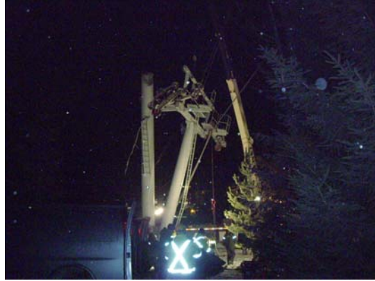
View of upper section of Tower #4 supported by haul rope and communication line (crane in place to prepare for removal of upper tower section)
