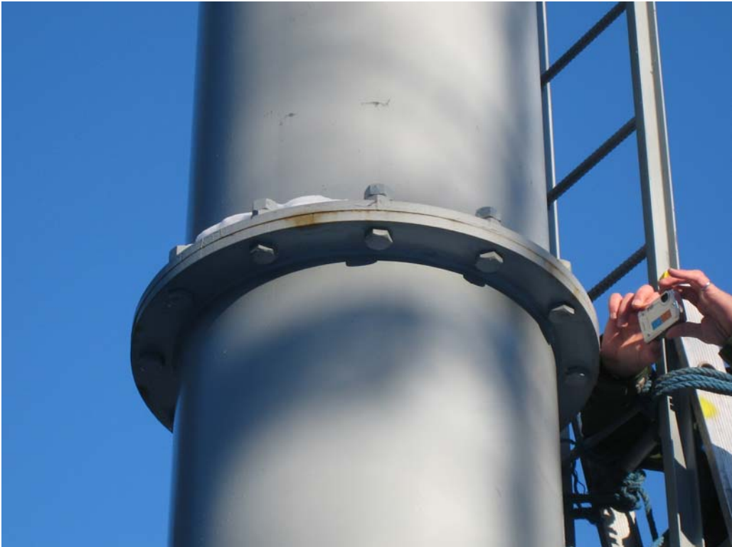
Lower Excalibur T5, rusted lower flange from water leakage
