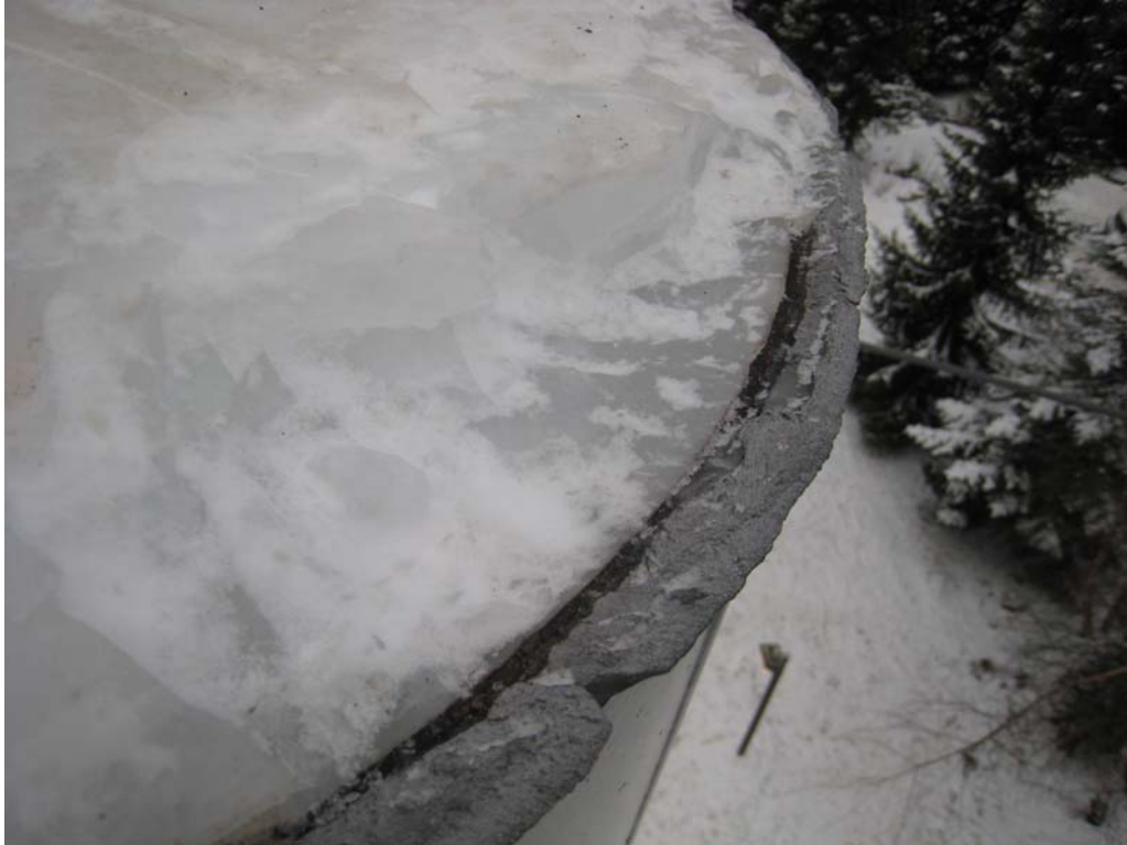
Lower Excalibur T4, incomplete penetration at lower section cap plate
