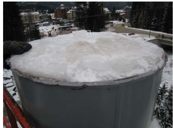
Top of Ice Column found in Tower #4 Lower Section Tube
