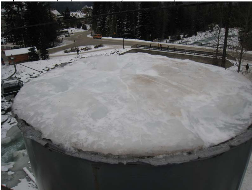
Lower Excalibur T4, Ice protruding above failed connection
