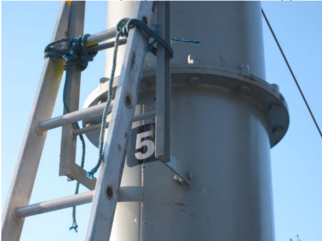
Lower Excalibur T5, pilot holes to determine concrete/ice interface
