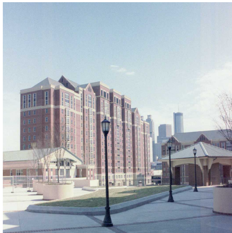
Figure 4. Completed Dormitory Building B in GSU Complex
