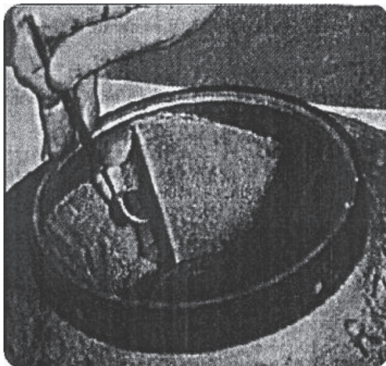
Figure 5: Examining the pressure side of the inlet vanes for suction recirculation.
