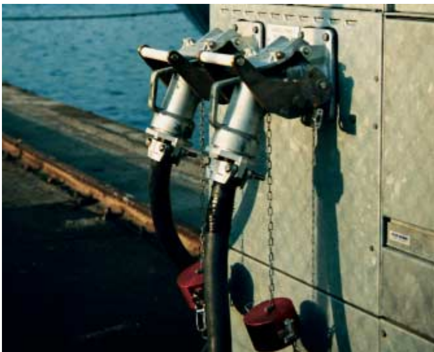
Above two X-type connectors in the harbour of Stockholm. The unique Push & Pull design assists the operators to connect the plug and socket without effort.
