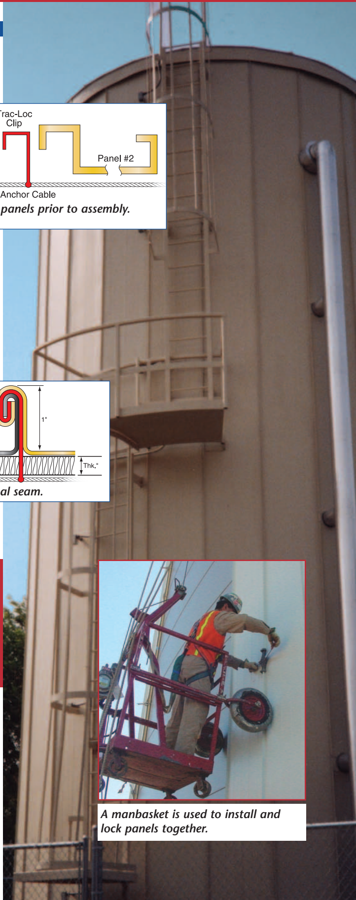
A Trac-Loc clip secures the panel to the cable.
