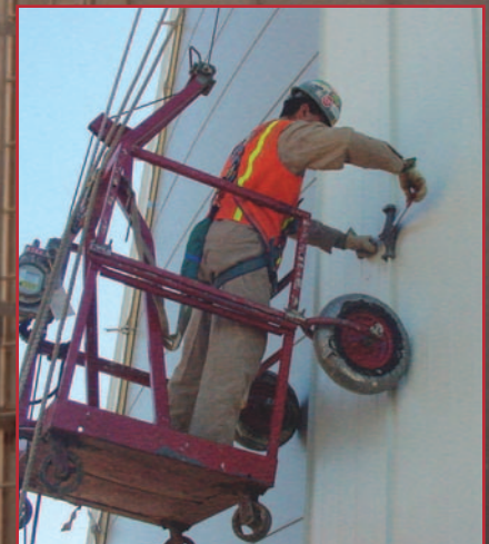
A manbasket is used to install and lock panels together.
