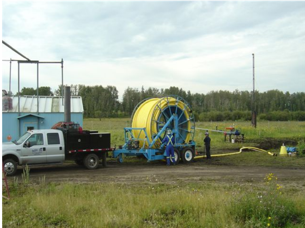
Figure 7-3 Spoolable Pipe Transport on Reel Trailer ( Photograph courtesy of Wellstream International Limited )
