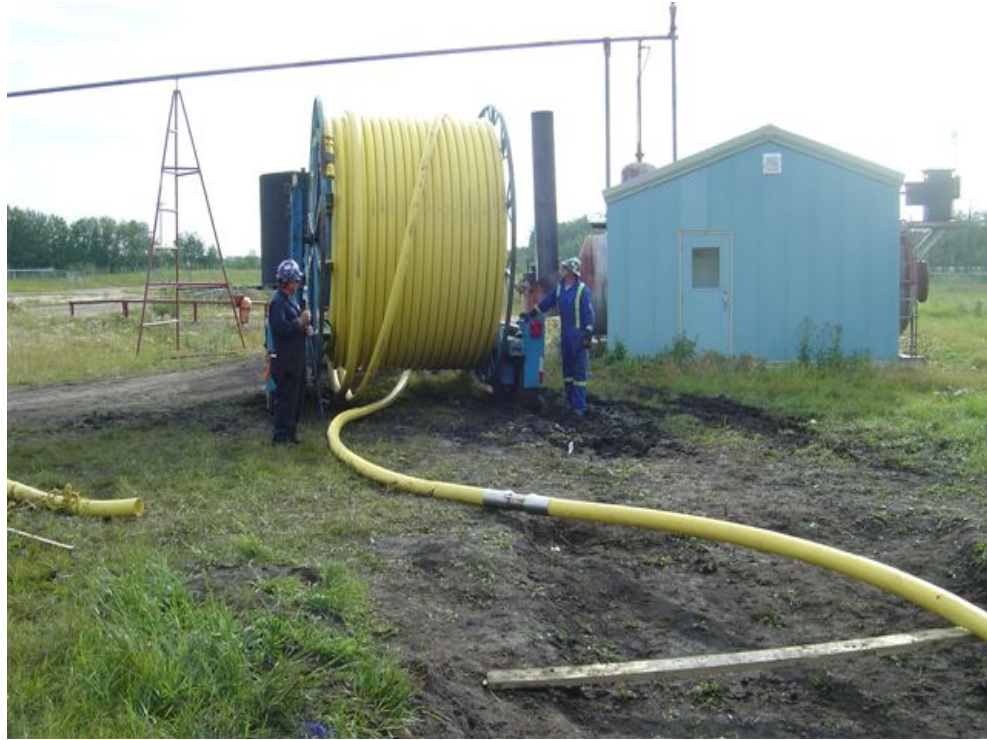
Figure 8-2 Metallic Coupler Joining Sections of Spoolable Pipe ( Photograph courtesy of Wellstream International Ltd )
