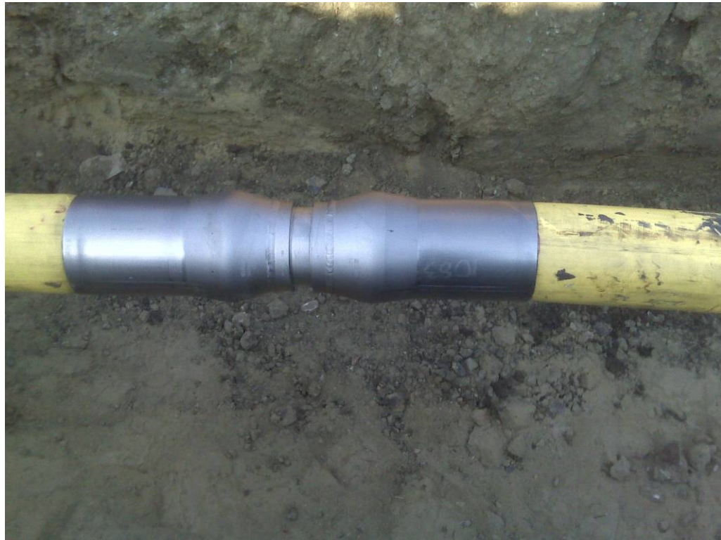
Figure 4-2 Spoolable Pipe Metallic Coupler Installation ( Photograph courtesy of Wellstream International Limited )
