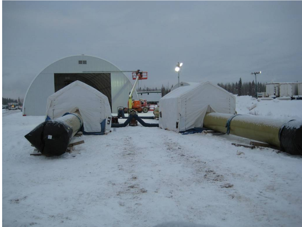
Figure 8-1 Provision of Shelters for Joining Composite Pipe; (Photograph courtesy of Fiber Glass Systems and Fiberglass Solutions Inc)
