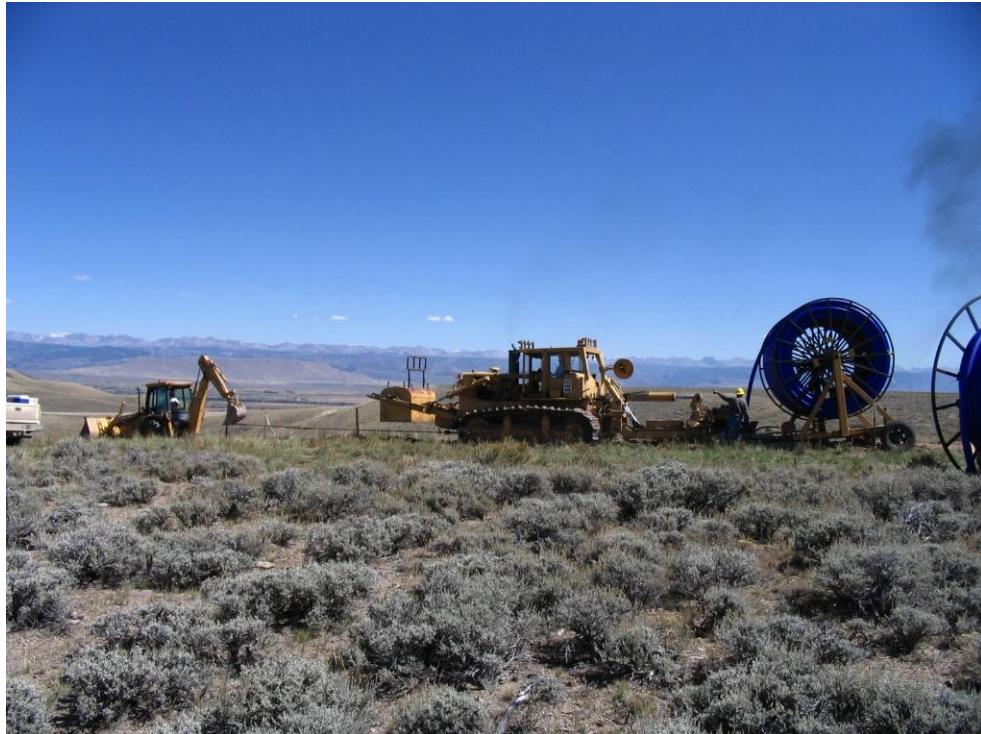
Figure 7-1 Typical Spoolable Reinforced Thermoplastic Pipe (RTP) Plough-In Installation Method ( Photograph courtesy of Flexpipe Systems )
