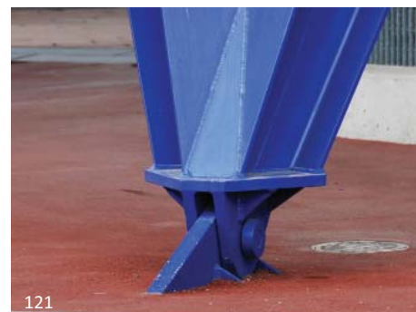
121 Good quality welding should require no special after-treatment (grinding) for the majority of AESS applications (Categories 1 through 3). Grinding would be considered only for Category 4 applications if a seamless appearance is important.
