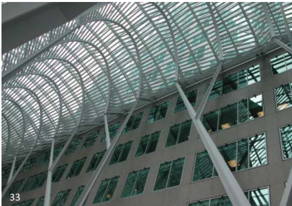
BCE Place in Toronto by Spanish Architect Santiago Calatrava uses AESS 4 quality fabrication and finish on the lower portion of the tree supports in the Galleria space. All of the members use welded connections with a hand-smooth finish and no apparent blemishes. Given the articulation and complicated geometry, tolerances for this structure were even less than one-half standard fabrication. The “canoes” that form the support for the skylight are well above view level and use a combination of welding and bolting.
