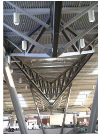
Ottawa International Airport: The steel trusses and sloped column supports are within view and touch by the passengers. The geometry of the steel is complex, and the tolerances and finish requirements are characteristic of AECS 3 Feature Element type steel.
