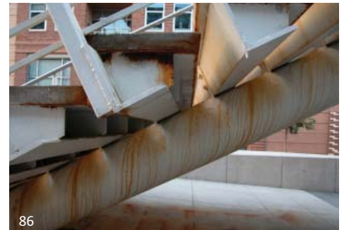
The white painted finish on this exposed steel exterior stair was not a good choice. Salt applied to the treads has resulted in rust stains on both the supporting steel and the concrete below.
