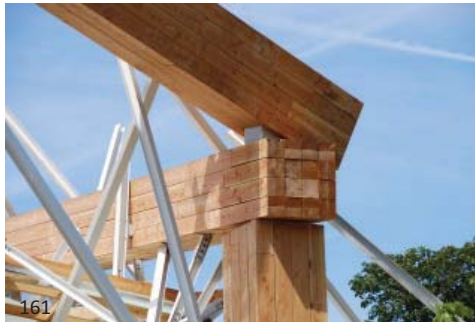
161 The heavy timber on this sculptural project is really “for show” as the main support system is all steel and the large square wood sections are used only to bulk out the form and provide a contrast with the steel used to support the glass.
