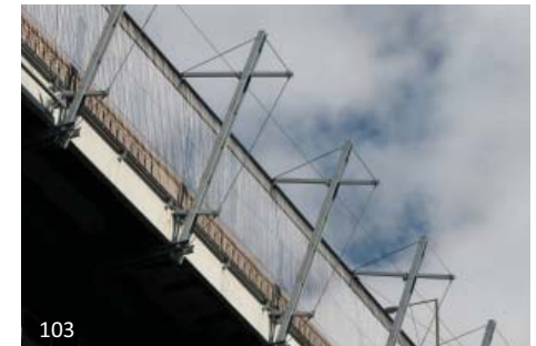
103 Galvanizing is a suitable finish for an exterior AESS structure that will be constantly subjected to weathering as in this expressive railing system.
