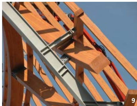
Composite structural systems require higher levels of coordination. The tolerances and construction practices of the other material must be taken into account.
