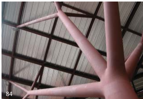
Extreme care and highly specialized detailing was required to join the branches of this tree to the casting nodes. Mechanical pipe was selected for its seamless appearance and structural properties. The surface had to be perfect given the application of a glossy painted finish and focus lighting.
