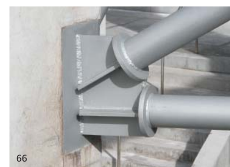
Fig. 3.6B This design used all-welded connections, even for this anchoring detail of the truss to the base plate. Bolted connections were not desired.
