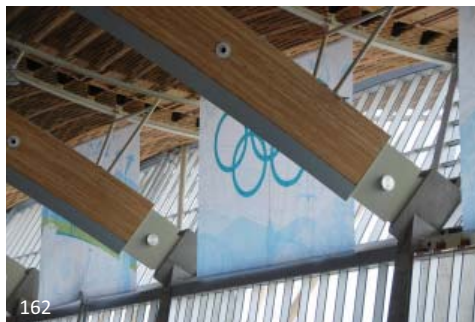
162 The large arches over the Richmond Speed Skating Oval are fabricated from a combination of steel and wood, with the majority of the steel hidden beneath the wood cladding of the arches.
