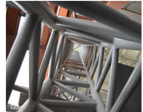
122 Although the overall form of this box truss appears complex, the 100% welded connections have been designed with simple geometries.
