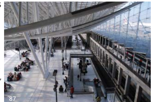
The painted white structure at the TGV Station at Charles de Gaulle Airport in Paris has proven difficult to keep clean. Access is not possible over the full width of the station, leading to severe buildup of grime over part of the structure. The structure is easily viewed from above, making the surface condition even more obvious.
