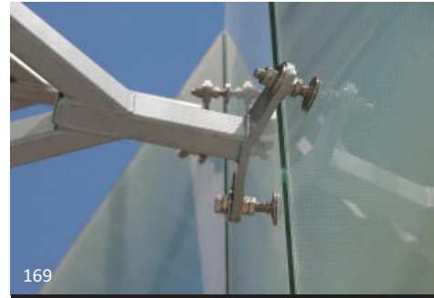
169 Alignment issues between the glass and steel support frame are taken care of by levelling mechanisms that are part of the glass connection system. These are located on the rear of the canopy and are not visible from the front, allowing for clean lines and uniformity on the public side of the system.
