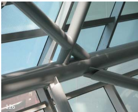
126 These tubular members were welded, using both tube-to-tube connections as well as X-shaped plate fabrications to resolve the geometry of the transition.
