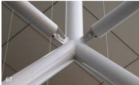
Fig. 4.1. This project uses mechanical pipe instead of HSS, as the three-dimensional nature of the structure made positioning seams out of view difficult, and a seamless appearance was important. Grinding of the seams would have been prohibitively expensive as well as time-consuming.
