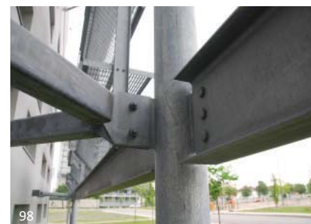
As can be seen in this galvanized exposed steel exterior shading system, a variety of finishes can be seen on the different hot dip galvanized members. This is to be expected in this sort of application.
