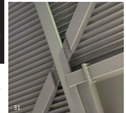
In the Canadian War Museum there are exposed welded and bolted connections. Square plates have been welded to the HSS members that provide surface for bolts on all sides of the connection to ensure a uniform appearance. Flat plates have been used for the lap-type hinge connections on the diagonal members, creating a degree of uniformity within the scheme.
