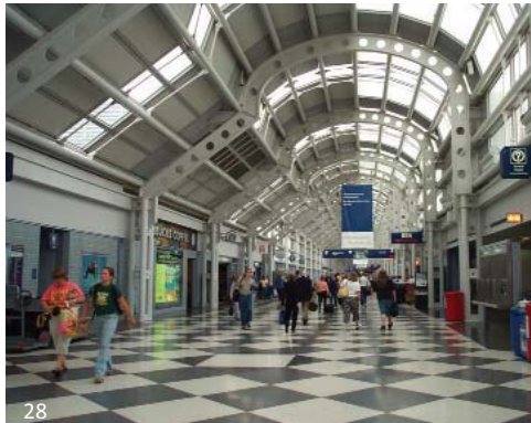
O'Hare International Airport in Chicago was the first airport to use AECS. Much of the steel is well within range of view and touch. A variety of steel shapes and connection types have been used. The complex nature of the sections and connections called for a tighter sizing tolerance and even finish application.
