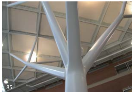
Extreme care and highly specialized detailing was required to join the branches of this tree to the casting nodes. Mechanical pipe was selected for its seamless appearance and structural properties. The surface had to be perfect given the application of a glossy painted finish and focus lighting.
