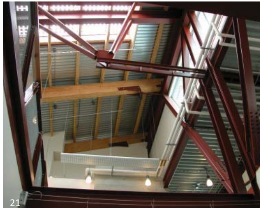
21 National Works, Vancouver B.C.: The project uses a more articulated steel design, predominantly with W-sections. Much of the structure is located at ceiling height, so at a distance for viewing and therefore allowing for a lower level of detailing and fine finish. This structure interacts with wood, which will change aspects of its detailing and coordination during erection.
