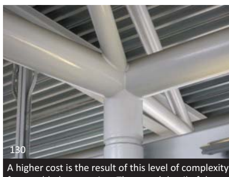
130 A higher cost is the result of this level of complexity for a welded connection. The reveal detail of the connection of the upper structure to the column makes the connection simpler to erect.
