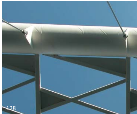
128 The large HSS members used on this bridge have helical welds. Although unusual in appearance, they were aesthetically worked into the design.
