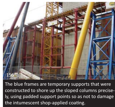
There was virtually no staging area at this busy downtown intersection, so the lifts all had to take place quickly at night. Hidden bolts were used on this seemingly all-welded structure to facilitate erection.
