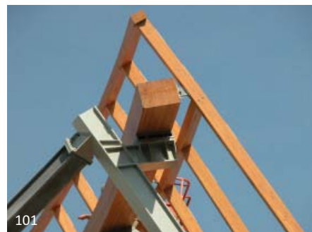
101 Here galvanized steel members are mixed with zinc painted grey steel. It was decided not to galvanize some of the members due to the chance of deformation in the hot zinc bath and potential stress release of the welds.
