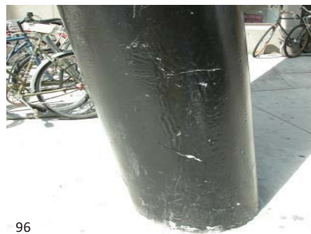
This thick intumescent coating is constantly being repaired due to its high traffic location as well as repeated incidences of graffiti removal. The colour matching on some of the supports is more difficult to achieve.
