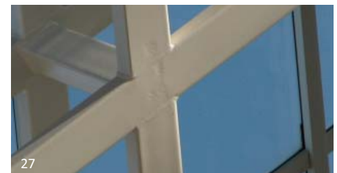
25 Edmonton City Hall: The trusses that support the pyramidal glass roof are created using square HSS sections. The viewing distance varies but is typically greater than 6 metres, even from the upper levels. An up-close inspection reveals many inconsistencies that are reasonable to leave “as is” due to the view distance. The extra expense to fill, grind and carefully align the members would be lost on users of the building.
