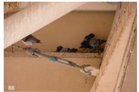
Ledges provide an excellent roosting place for pigeons. Remember to install pigeon-deterrent fences and surfaces to prevent roosting and the associated soiling of the structure and spaces below.
