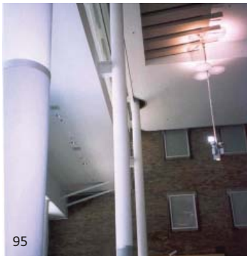
The colour and texture of intumescent coatings are not the same as normal paint, so it is necessary to detail items like these columns to recognize that the finishes are not the same. Here a band of a different colour highlights the change.
