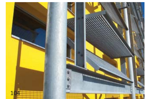
104 Galvanizing is very popular as a finish, but remember that its basic purpose is as a corrosion-prevention coating. The nature of the finish will not be consistent from batch to batch.
