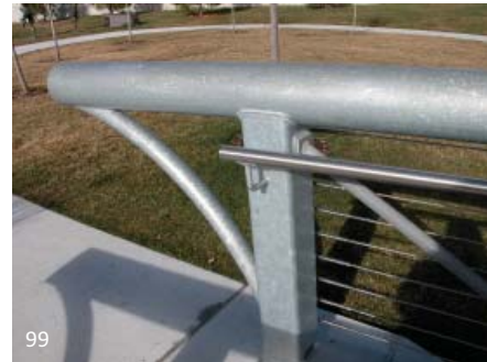
99 Seal welds have been used to connect the various components of this exterior galvanized steel feature railing. There is a large opening at the base of the square HSS post to allow any water that may enter the railing an opportunity to drain.
