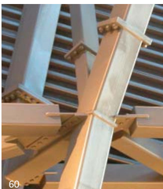
Fig. 3.3B The seams on the square HSS sections have been aligned and, even on the outside face of the connection, seem in keeping with the overall design intention.
