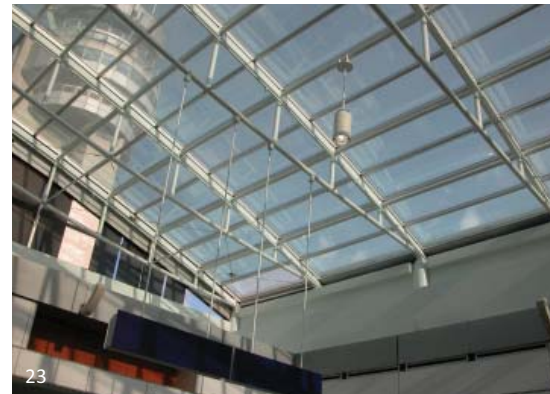
23 Pierre Elliott Trudeau Airport, Montreal: The trusses supporting this skylight are quite characteristic of AESS 2 type steel. The viewing distance is over 6 metres but the design needs something more than a standard joist or truss. The detailing is simple, and the viewer is not close enough to see the texture of the connection, only the form of the truss.
