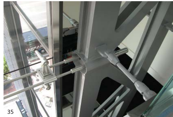
The Newseum in Washington, D.C. by Polshek Partnership uses a combination of AESS 4 quality steel with some custom specialty elements in this inventive support system which forms the support and wind bracing for a large mullionless glazed wall at the front of the building. Stainless steel brackets hook on to parallel tension supports that are braced on either side of the façade by these vertical trusses fabricated from parallel sections of plate steel.
