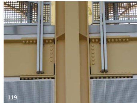
119 The aesthetic of this project included a high level of texture using standard structural shapes, and so bolting was chosen.
