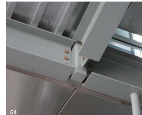
Fig. 3.5B This exposed bolted connection is tightly designed and demonstrates uniformity in the joint gaps.
