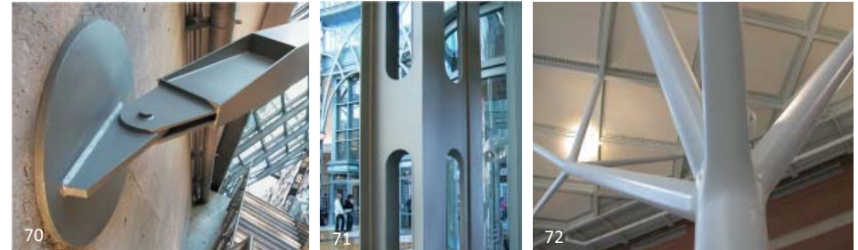
Fig. 4.3B Surfaces filled and sanded. These three examples show very different applications of AESS 4 whose details require extra care and high-level consistency such that any and all imperfections are filled (typically with body filler) and sanded prior to the application of the finish coating. It is particularly important in the left and right images where a glossy finish is to be applied.
