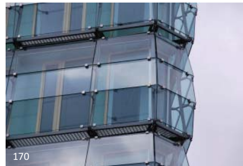
170 The steel supports for this double façade envelope use a system of clips to support the extra layer of glass. This alleviates issues of drilling of the glass and allows for better accommodation of differential movement between the systems.
