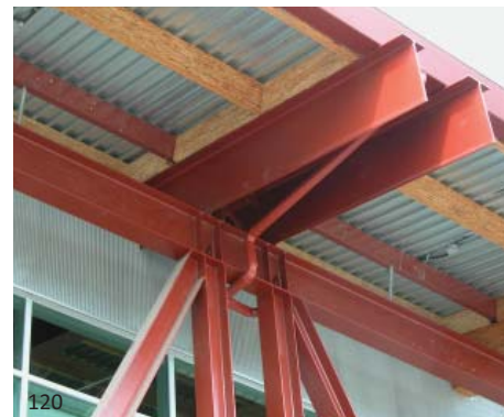
120 Welded connections have been used here in conjunction with the selection of W-members to create a very technical feel for the Works Yard.
