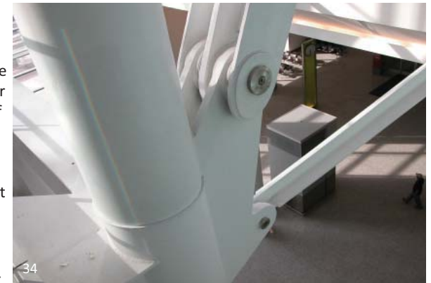
Pearson International Airport in Toronto uses a combination of AESS 4 for the columns and supports that are visible in the pedestrian areas, and Custom for the “wishbones” that form the supports for the roof trusses. The supports make use of more standardized shapes where the “wishbones” require significantly more effort on the part of the fabricator in the creation of specialty sections from plate steel.
