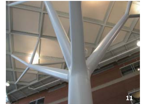
Two different steel trees: one created using W shapes to create a very textured appearance; the other using mechanical pipe and specialty casting and striving for a seamless appearance using a high gloss finish. AEES specifications must be tailored to the overall design intentions of each individual project as they are all somewhat unique.
