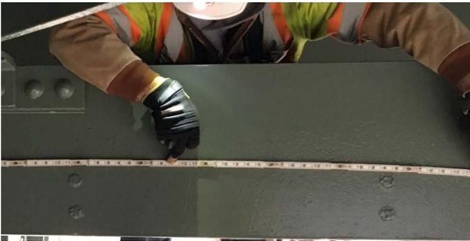
Figure 9 Tack-welded rivet shanks, member U19-19', near PP20 (HNTB)
