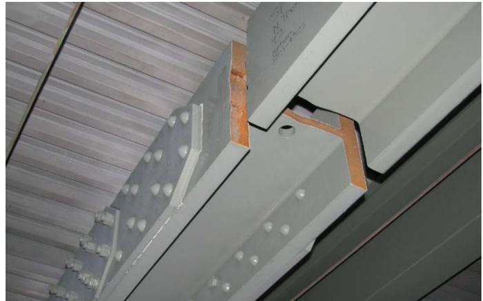
Figure 3 Fracture of U19-19', North Truss, Looking South and East at Panel Point 19', prior to any material sampling. (HNTB)
