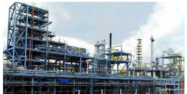
EUROPE - 48 MTPD H 2 S Production Facility. Licensed & Engineered by Unitel Technologies. Photo used with permission
