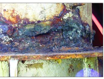
Effects of corrosion under insulation near angles on steel
