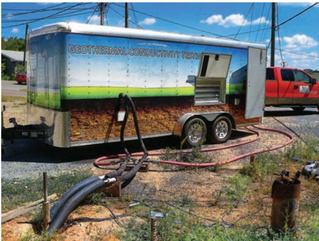
Figure 5. Field thermal conductivity test in progress.
