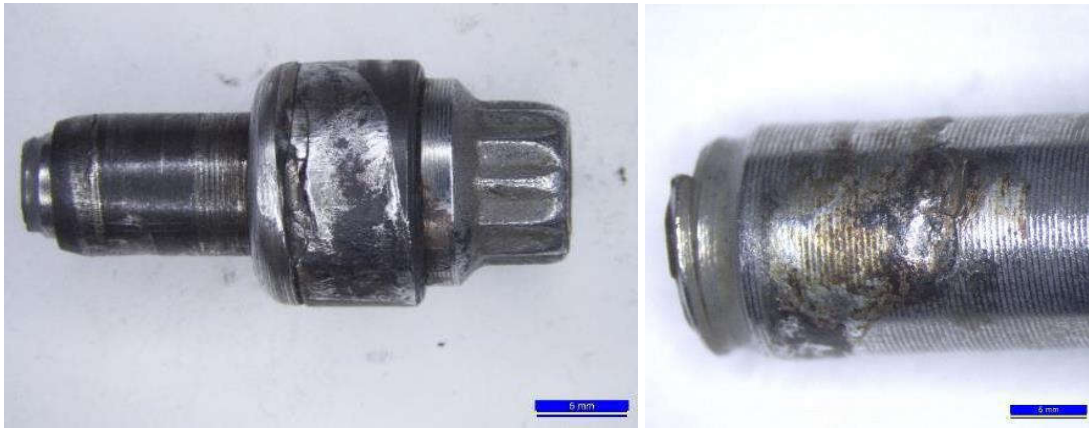
Figure 13 - Mechanical damage and cracking of the bolt collar (left) and fretting damage along the shank of the bolt (right)
