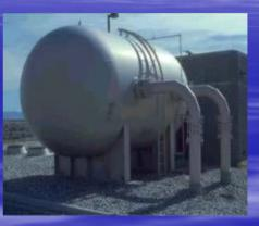
There are two types of gas accumulator used for the mitigation of surge pressures. Firstly there is a pressure vessel with a back up compressor that maintains the volume of gas in the unit to cater for pressure changes. The second is a pressure vessels fitted with an elastomeric bladder with gas one side and the process fluid the other. Shown in the previous slide.
