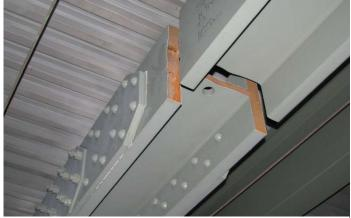
Figure 3 Fracture of U19-19', North Truss, Looking South and East at Panel Point 19', prior to any material sampling. (HNTB)
