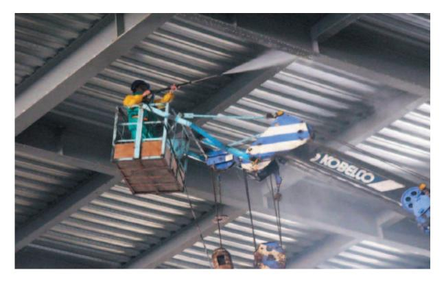
Figure 10: Intumescent paint being applied in the field
