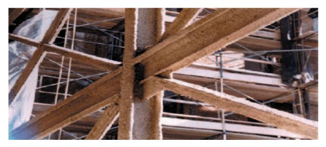
Figure 5: Conventional spray applied fire protection material
