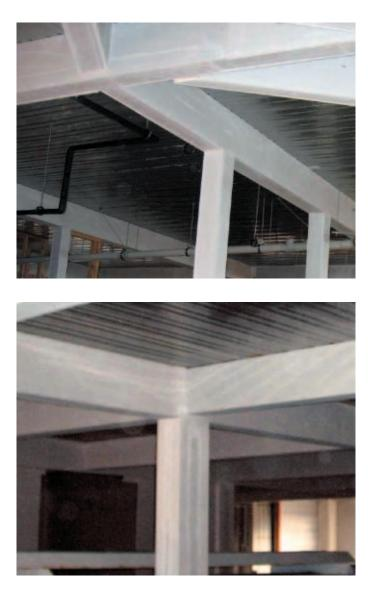
Figure 7 and 8: Steel sections clad in fire proofing board materials
