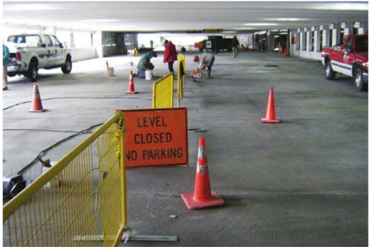
Maintenance and repair of deck connections is a common problem with precast double-tee garage construction.
