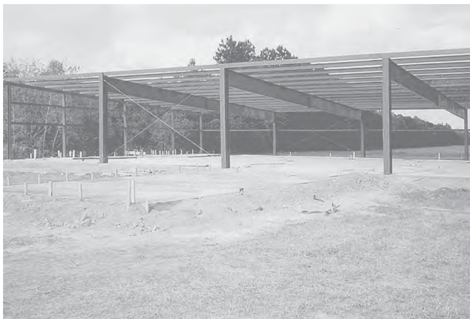
The portal method of analysis can be used to (approximately) perform a lateral-load analysis of this single-story frame.
