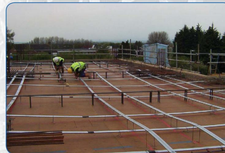
Fig 1 – decking painted to indicate tendon position
