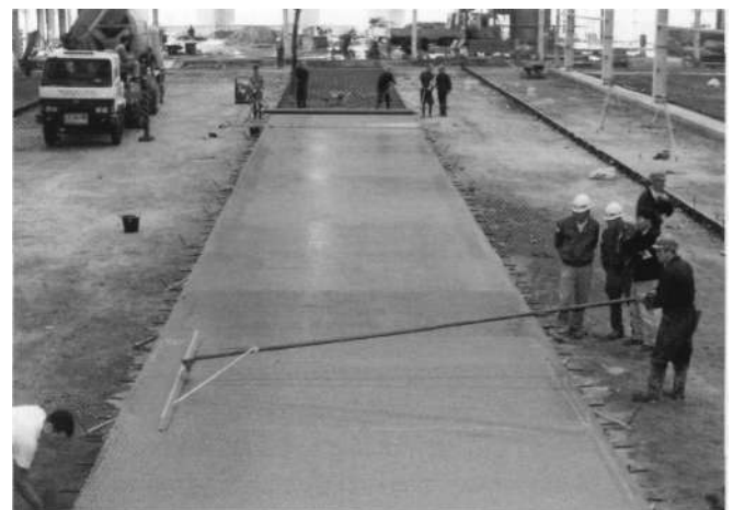
Figure 2.3: Long strip construction, allowing access for levelling using a highway straightedge.
