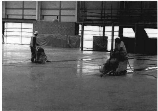
Figure 8.8: Joint sawing.
