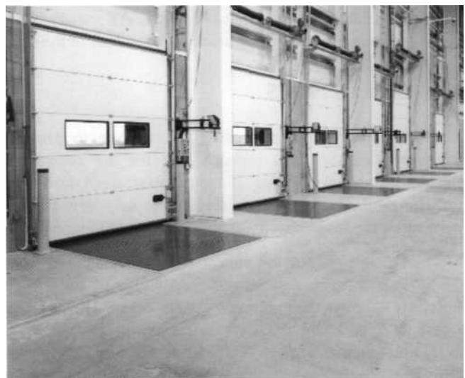
Figure 7.1: Dock levellers. Additional reinforcement may be needed in the areas around each entrance.
