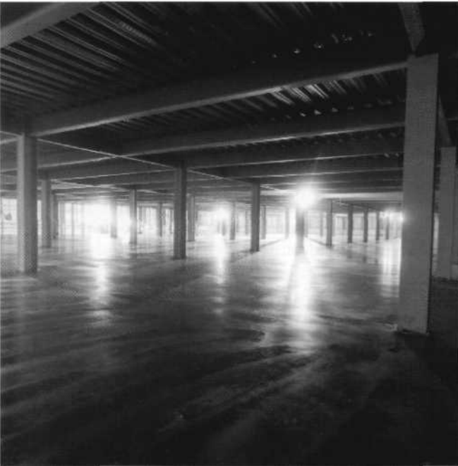
Figure 12.2: Successfully completed floor.
