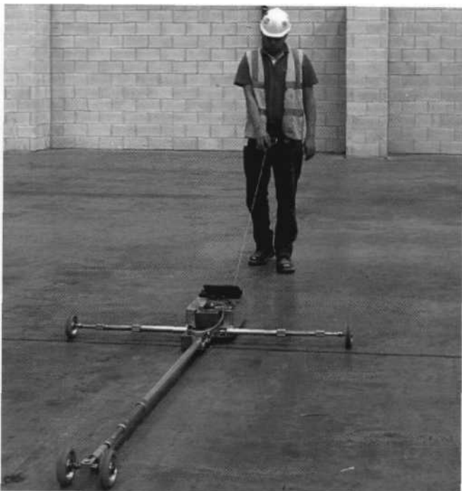
Figure C2: Surveying a defined-movement area with a profileograph prior to installation of racking
