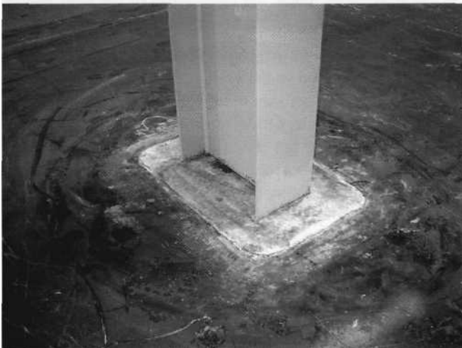
Figure 8.6: Isolation details around column.
