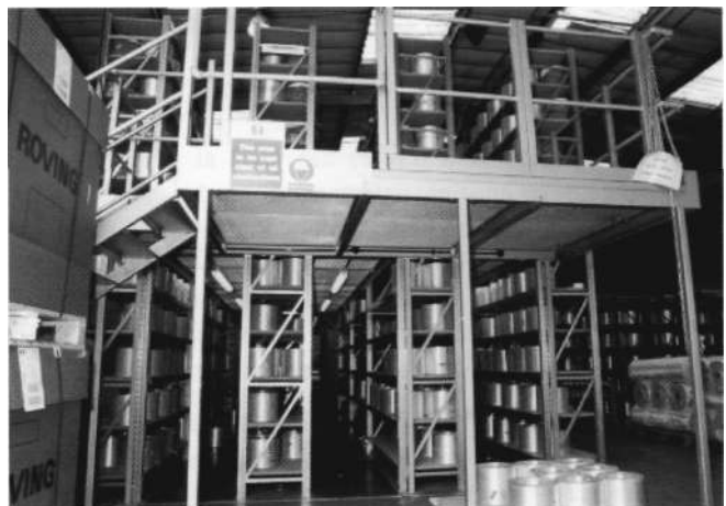
Figure 3.11: Mezzanine used for access to storage, with racking below.
