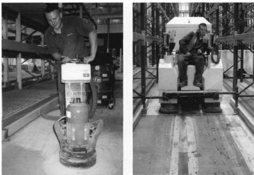
Figure 4.10: Typical grinding operations.
