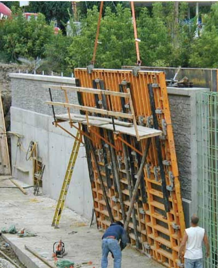
**Fig. 4:** Concrete wall cast using a formliner designed to simulate a masonry wall (photo courtesy of Gewalt Hamilton Associates)
