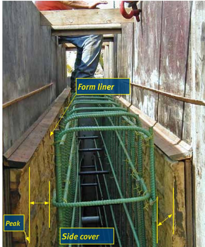
**Fig. 5:** View of formwork, formliner, and reinforcing showing side cover measured to the peak of the formliner
