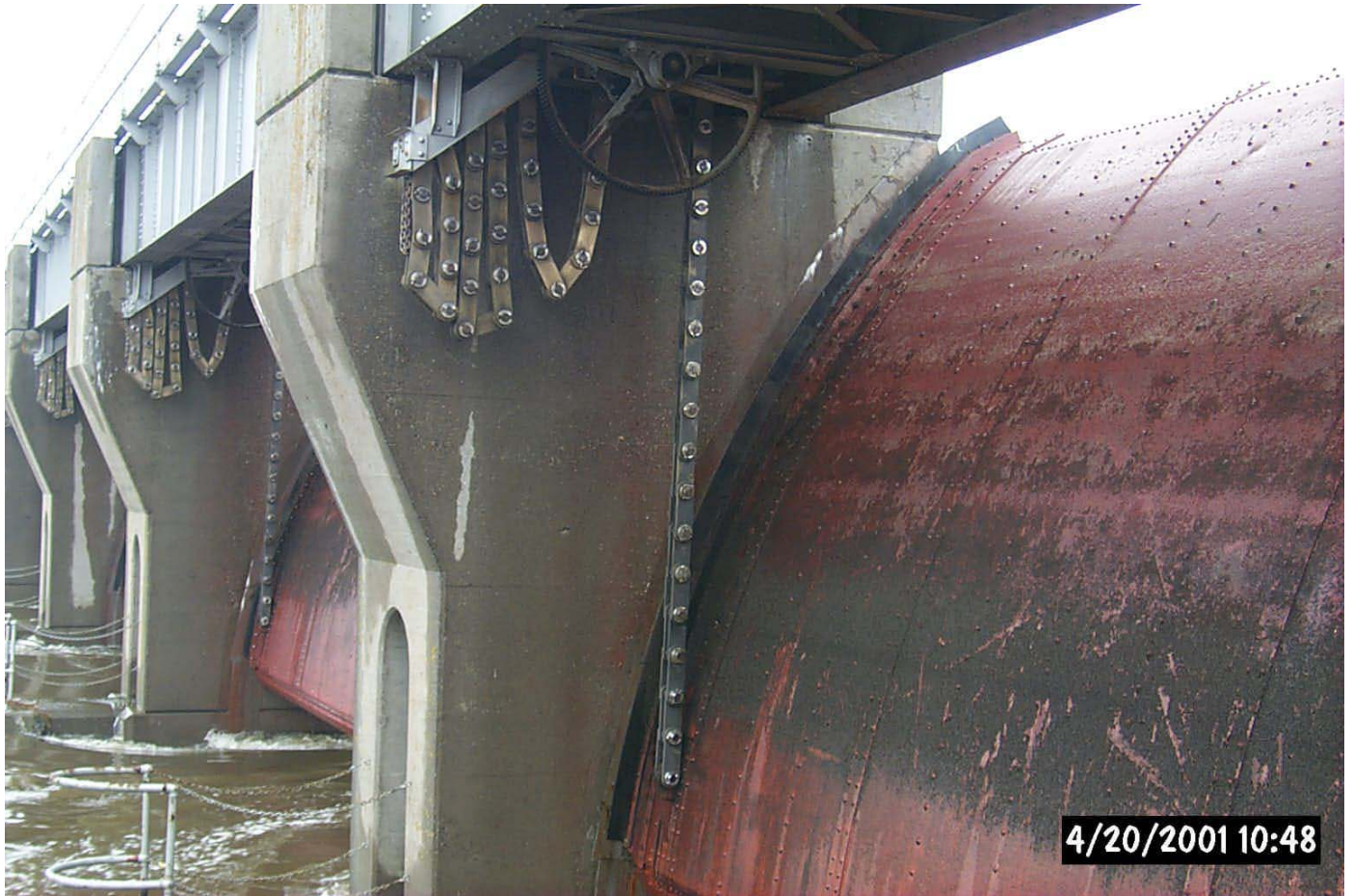
TYPICAL TAINTER GATE CHAIN INSTALLATION
