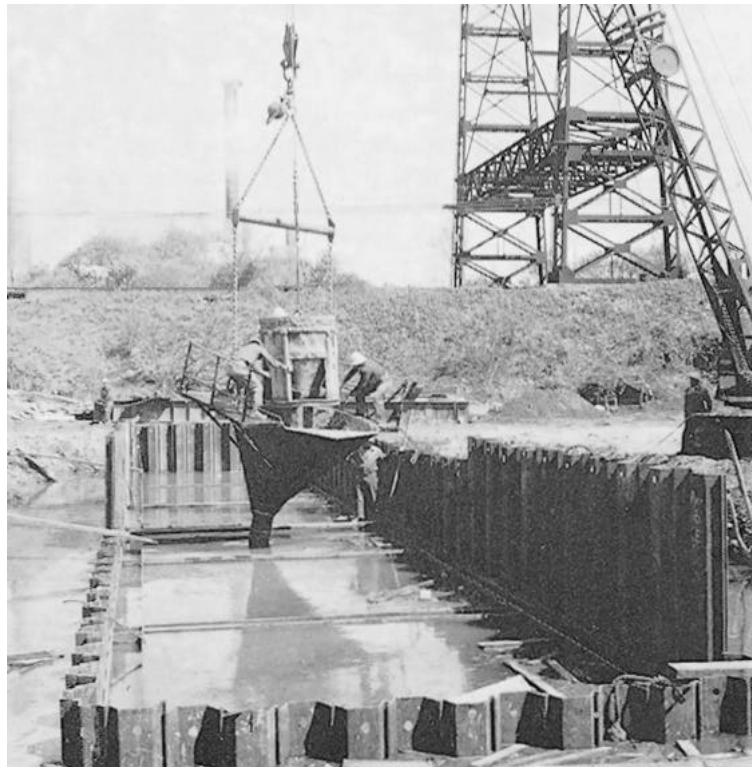
Placing tremie concrete for a bridge on the Connecticut Turnpike.
