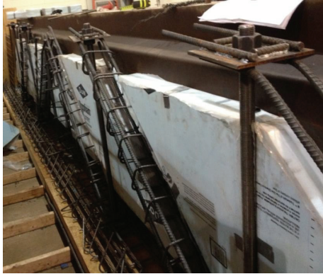
FIGURE 9: All reinforcements after being installed in the form.
