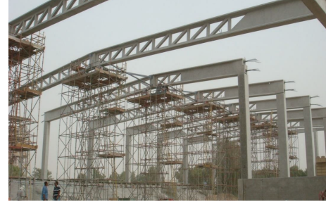
FIGURE 1: The temporary supports used before posttensioning (courtesy of e.Construct, LLC).
