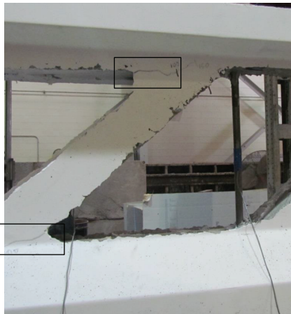
FIGURE 12: First cracks observed at 445 kN (100 kip).
