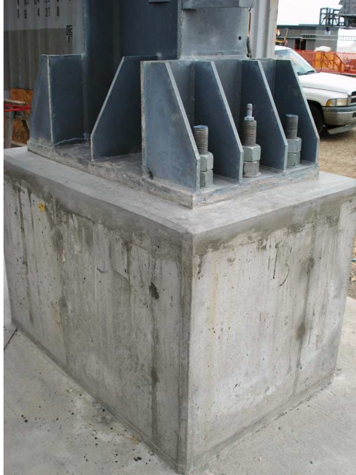
Figure 1. Pedestal supporting a compressor-building column
