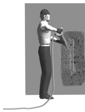
Unsound concrete removed with 15-lb chipping hammer. Hammers larger than a 15-lb class may cause damage to substrate and reinforcement.
