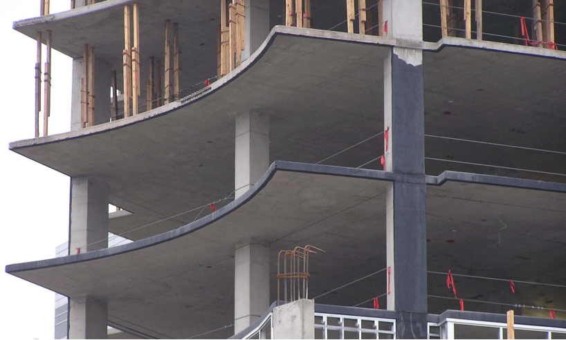
Figure 1.2: Flat Plate Reinforced Concrete Residential Structure Under Construction
