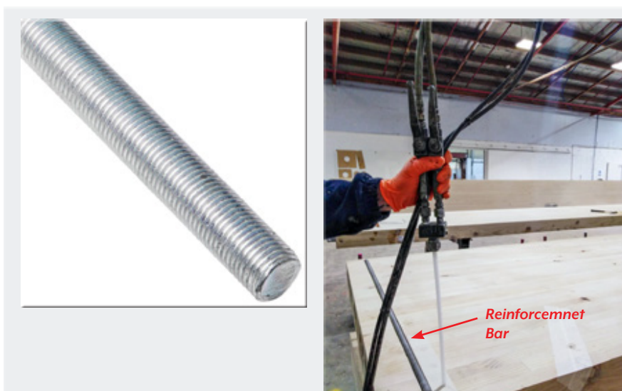
Figure 13: Reinforcement with fully threaded screws.
