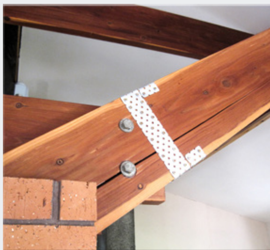
Reinforcement with a nailon plate (c/o Andy Buchanan).
