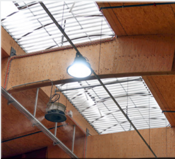
Figure 19: Reinforcement of curved beams with glued-on wood-based panels (c/o Robert Jockwer).
