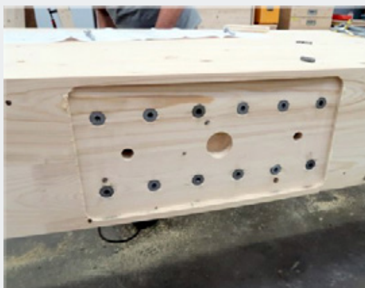
Bearing reinforcement with fully threaded screws and recess for a steel plate (c/o Robert Jockwer).
