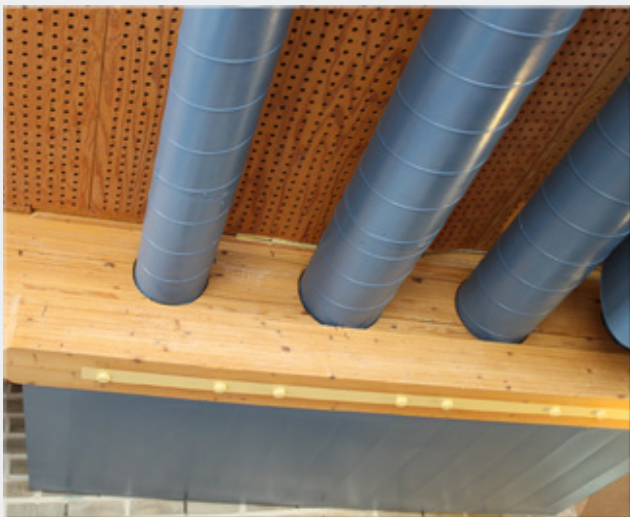
Reinforcement of penetrations with post-installed threaded rods (c/o Robert Jockwer).
