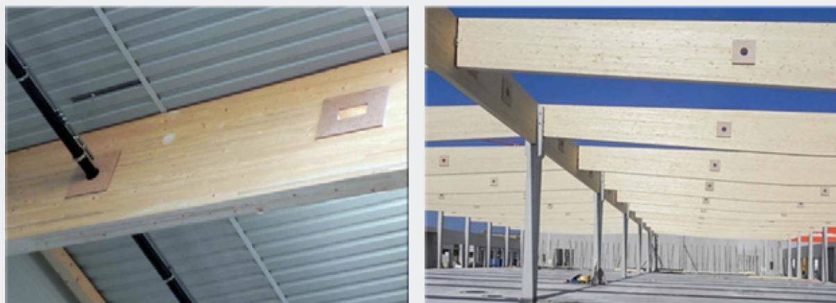
Figure 15: Reinforcement of penetrations with glued-on wood-based panels (c/o Wiehag).
