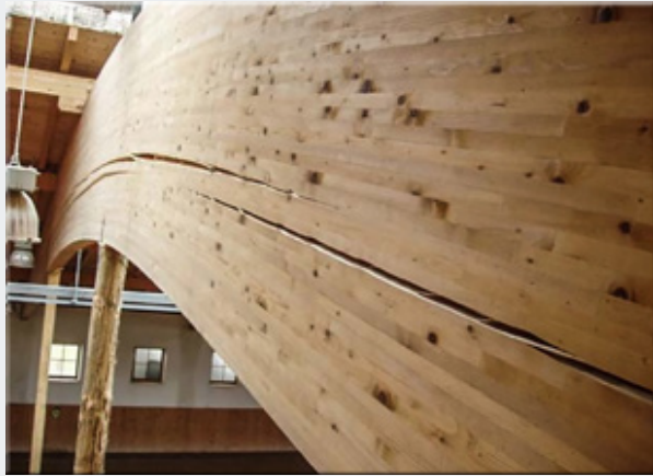
Figure 11: Splitting of curved and pitched-cambered beams.
