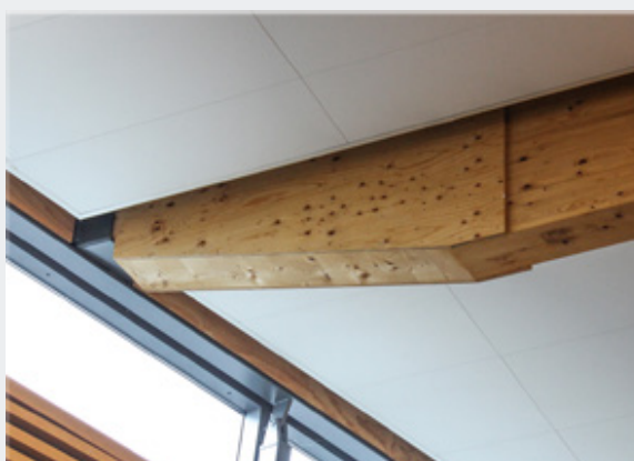
Reinforcement of a tapered notch with glued-on wood-based panels.
