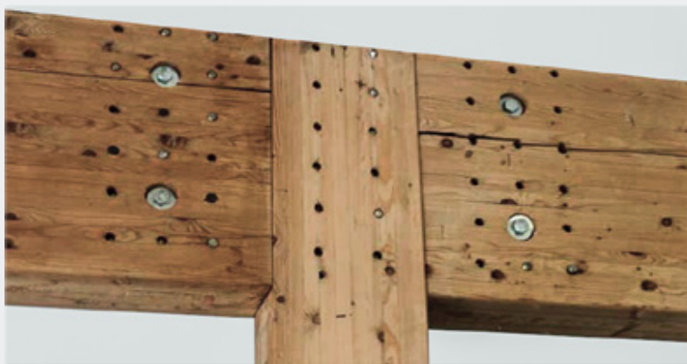
Figure 9: Splitting due to shrinkage restrained by steel plates (Brunauer, 2017).
