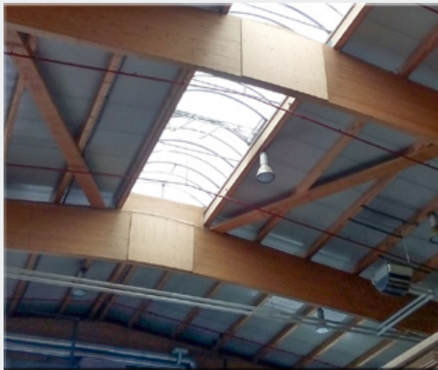
Figure 19: Reinforcement of curved beams with glued-on wood-based panels (c/o Robert Jockwer).
