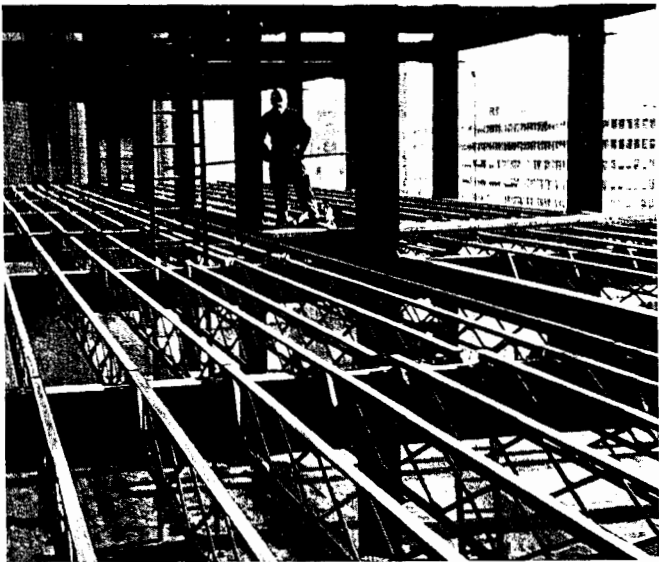
Bethlehem Joists arrive at the job site ready for placing.
