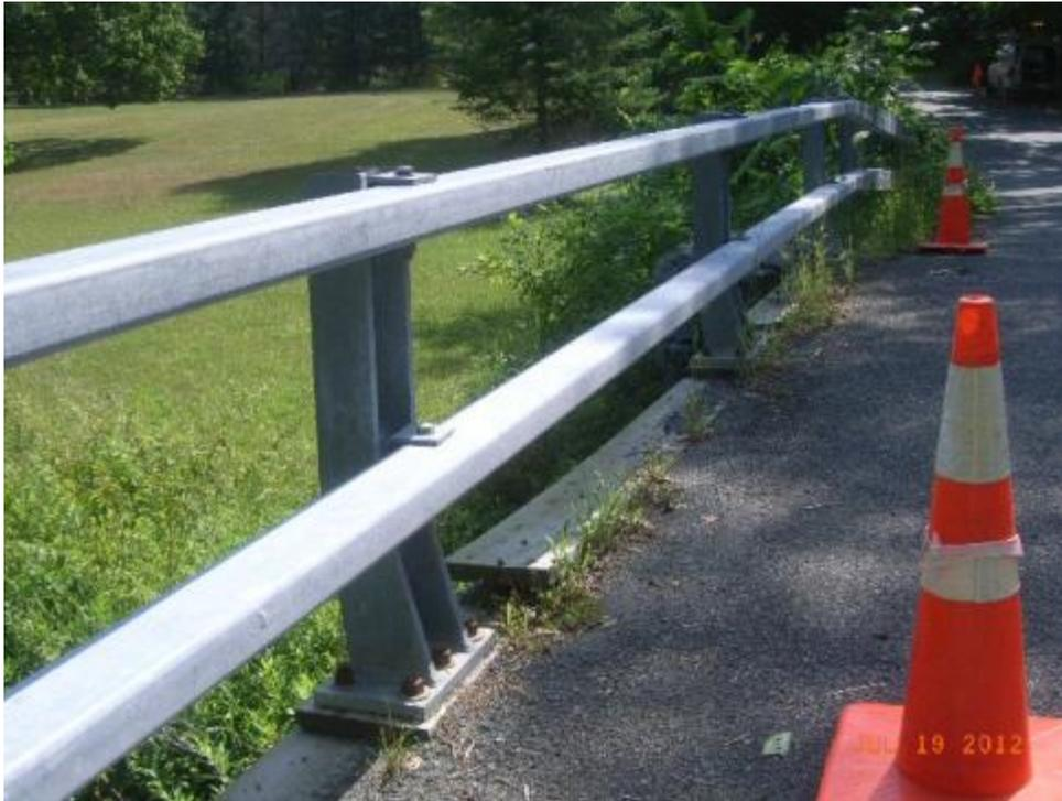
**Base plates directly on top of timber deck and through bolt with individual bottom plate – limited engagement of deck planks**
