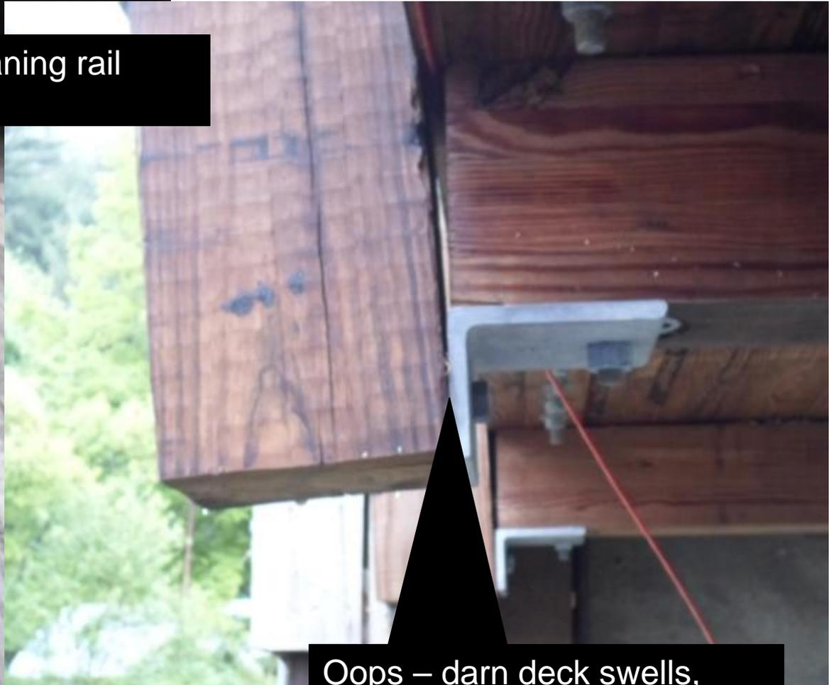
Oops – darn deck swells, more than the transverse stiffener – solution? – remove horizontal connection?
