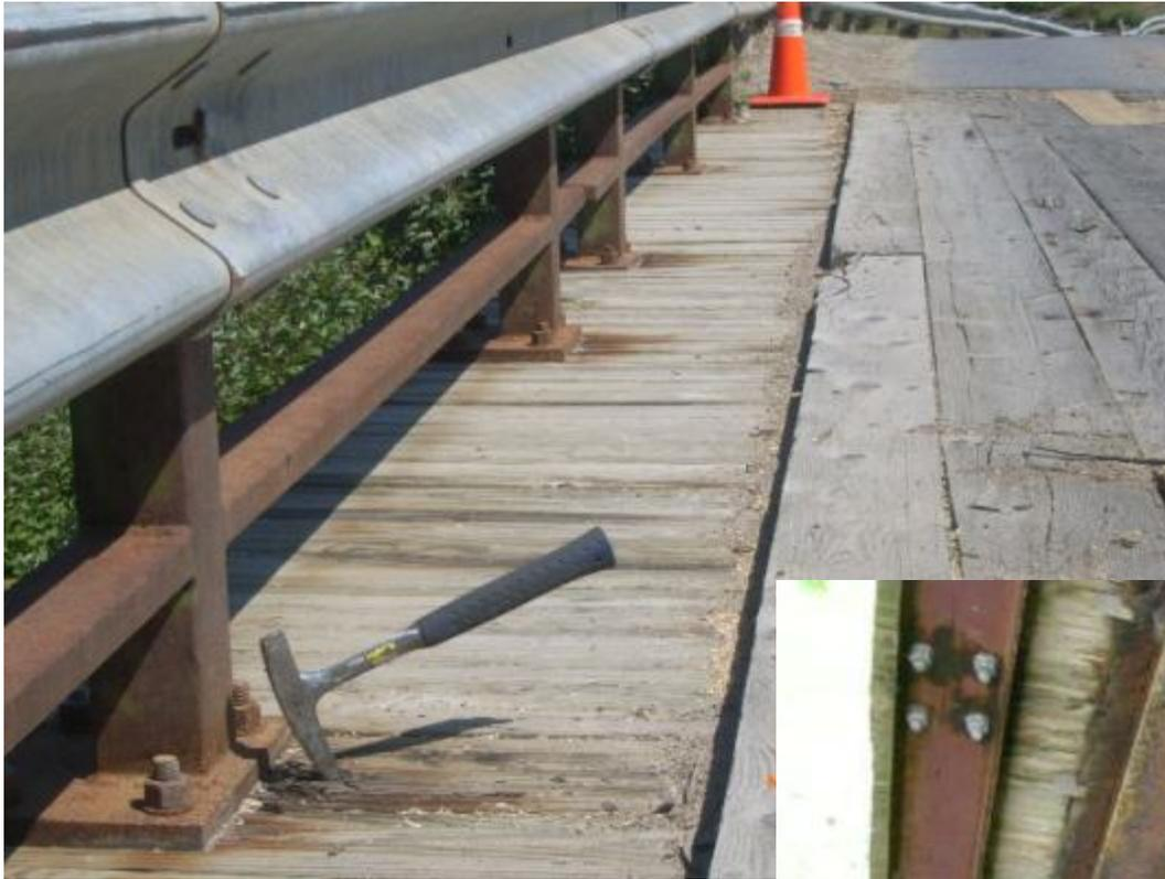
**Base plates directly on top of timber deck and through bolt with continuous channel on bottom – good engagement of deck**
