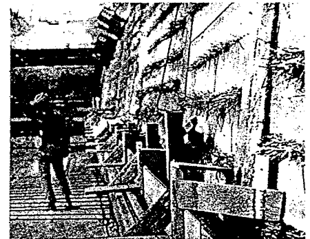
Fig. 2. Excavation here is 56 ft below ground level, yet design did not provide for keeping water in the sandy soil from entering excavation. Straw packed between wood lagging permits water to enter excavation, but prevents caving of sandy soil.
