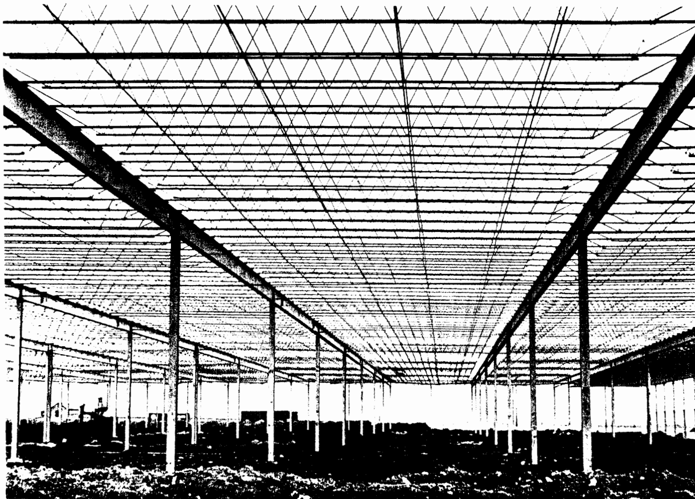
Typical joist installation by Berger Steel Company.
