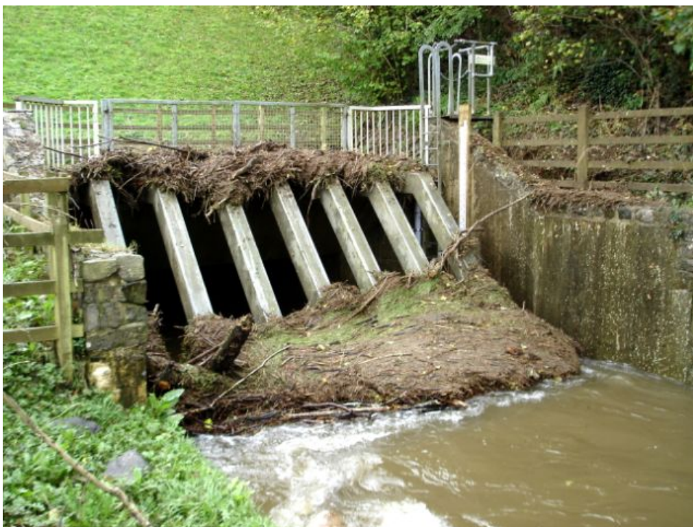
Figure 8.1 Coarse screen at a flood relief culvert inlet showing degree of debris build-up (the 'Beaverscreen' effect).
