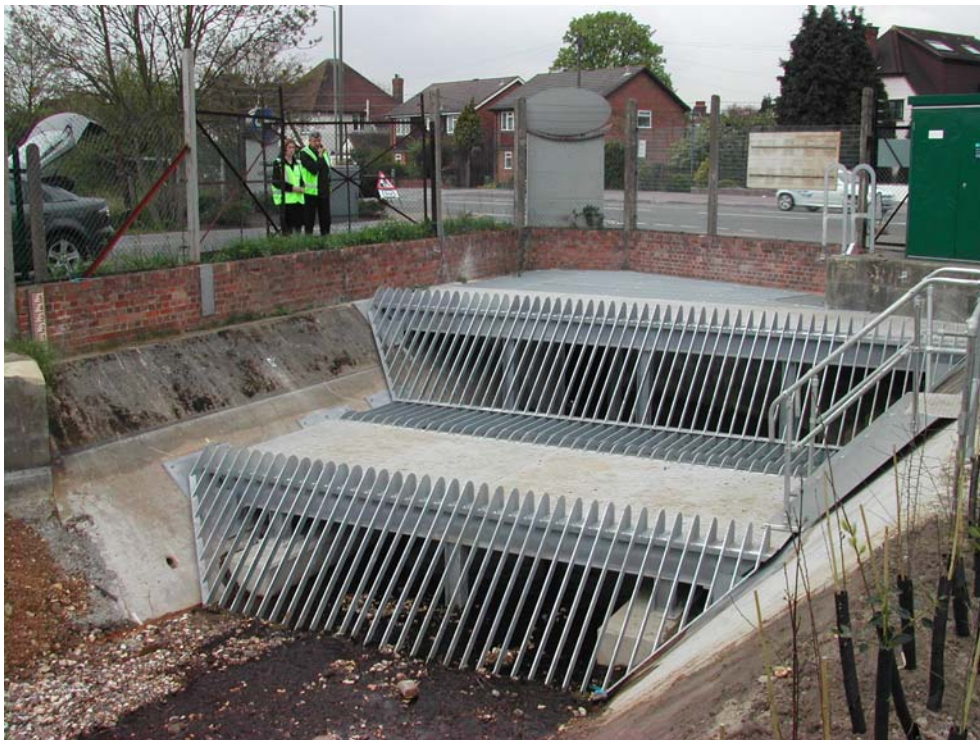
Figure 11.1 A recently installed screen in an urban setting.
