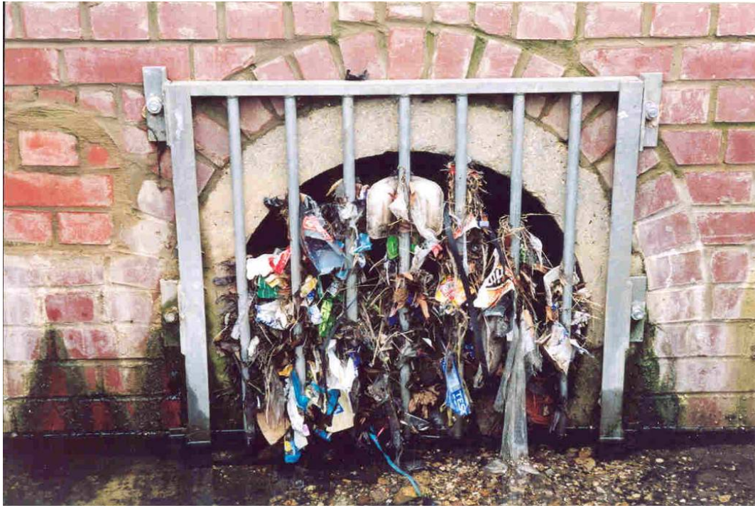
Figure 4.4 Crude security screen at the downstream end of a small culvert.
