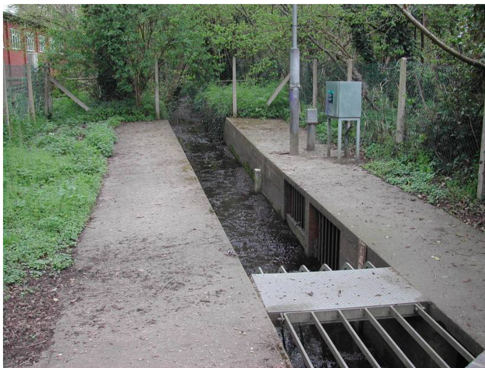
Figure 12.1 Kydbrook screen and bypass facility, Ravensbourne, South London.
