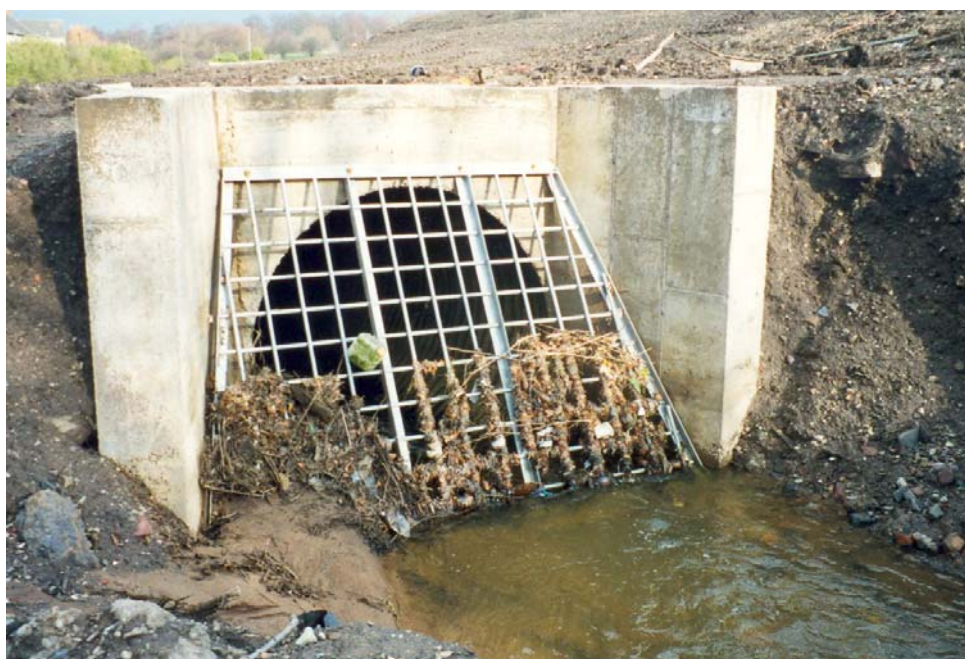
Figure 4.2 Poorly designed screen.
