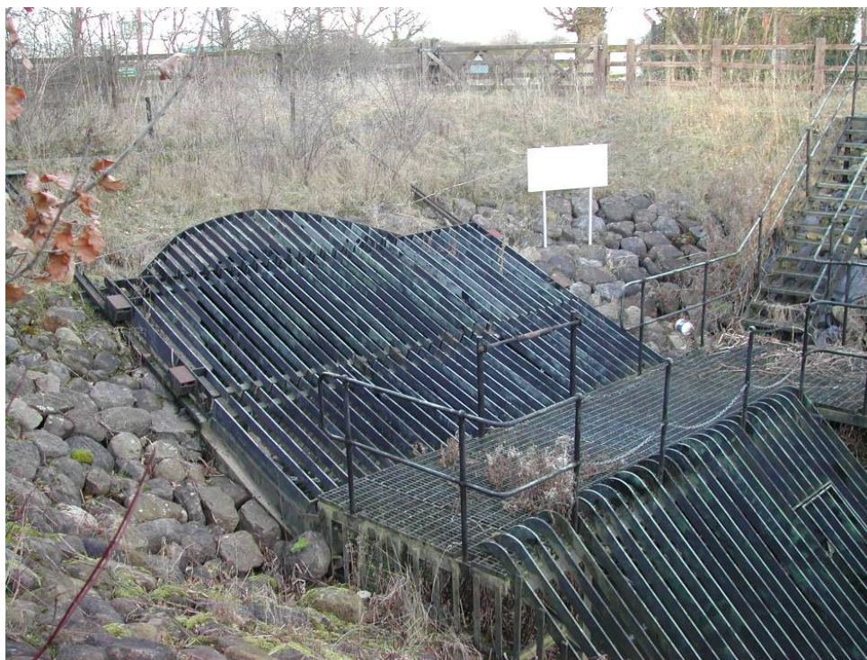
Figure 4.6 Security screen at the entrance to a large flood relief culvert.
