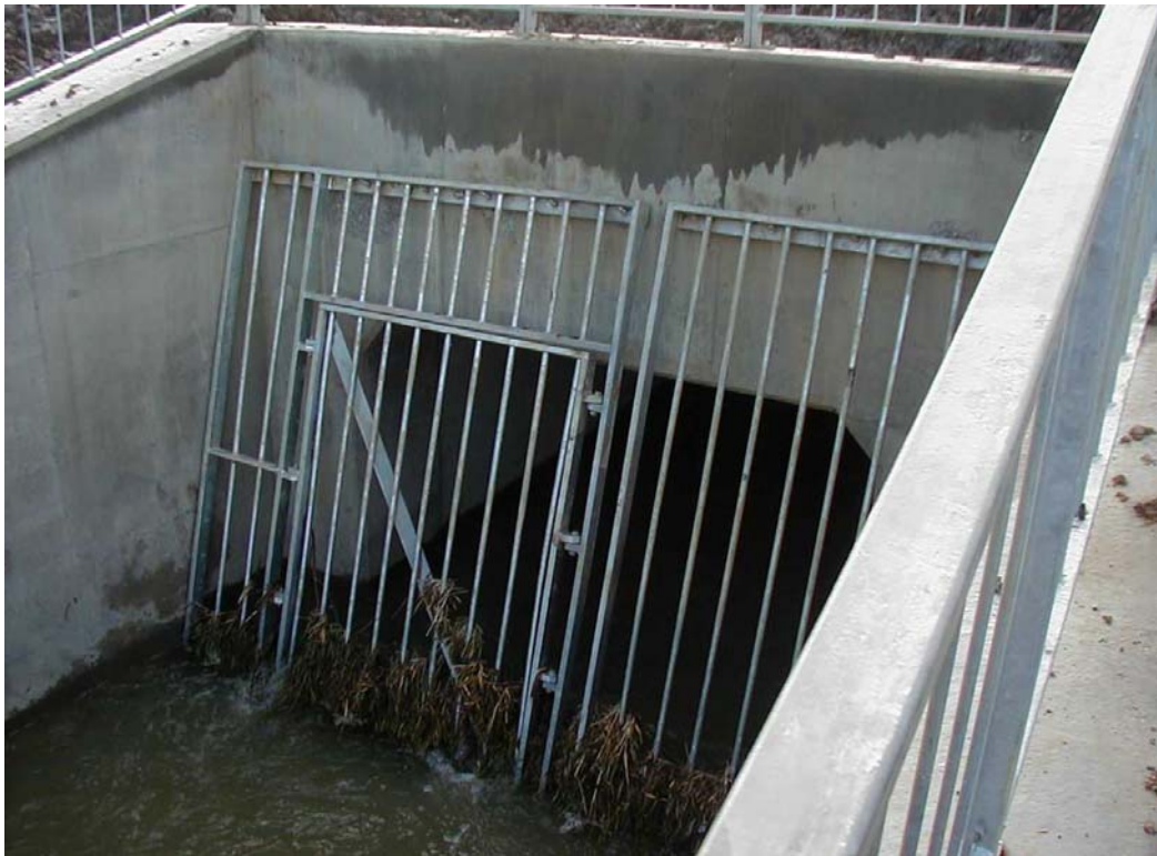
Figure 4.5 A security screen on the outlet of a culvert.
