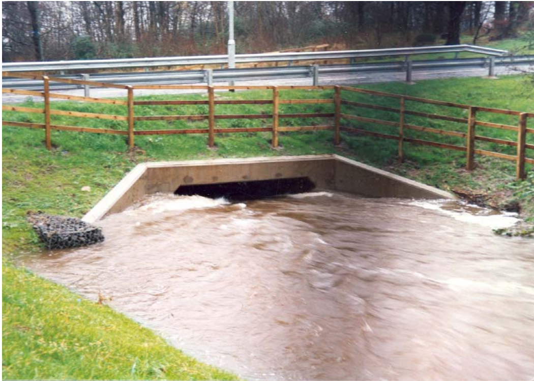
Figure 3.1 Highway culvert with no requirements for a screen.
