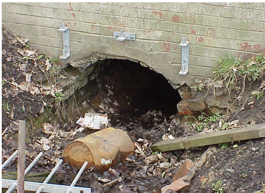
Figure 4.3 Screen on a small culvert not securely fixed in place.
