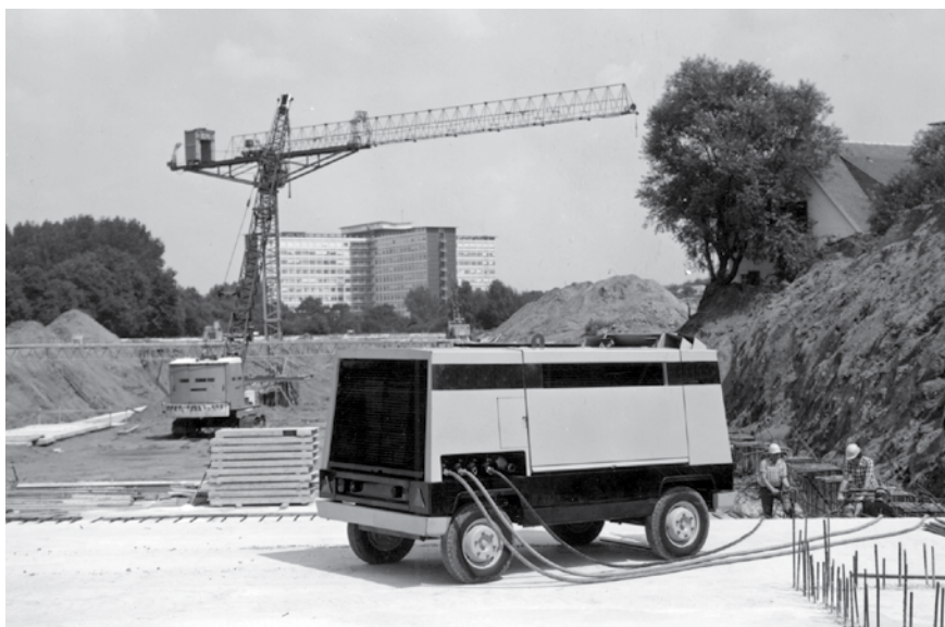
Figure 2.18 A 742 cfm portable compressor running several hand-held drills on a construction site.
