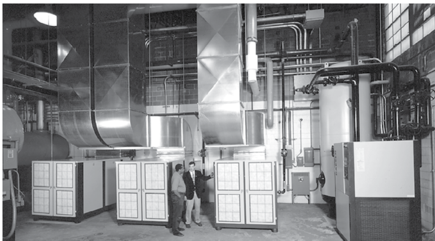
Figure 2.3 Installation of oil injected rotary screw compressors with heat recovery ducting.
