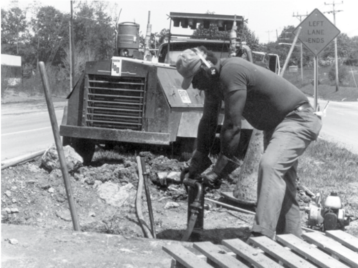
Figure 2.21 The drill on this air tool is working in rock six feet below ground level. The hole will accommodate the steel reinforced foundation for a highway sign. The compressor is a 100 cfm, 100 psig unit.
