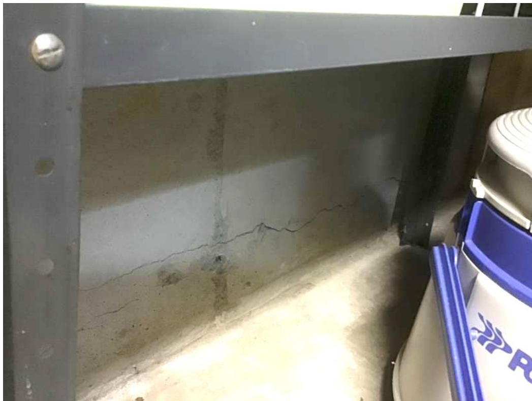
Bottom Crack
