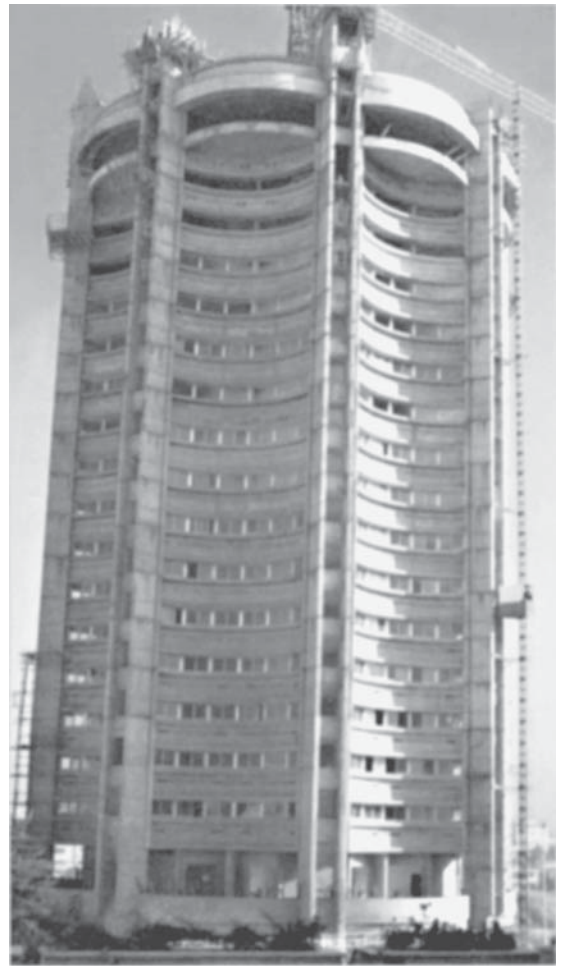
Curved beams in an office building.
