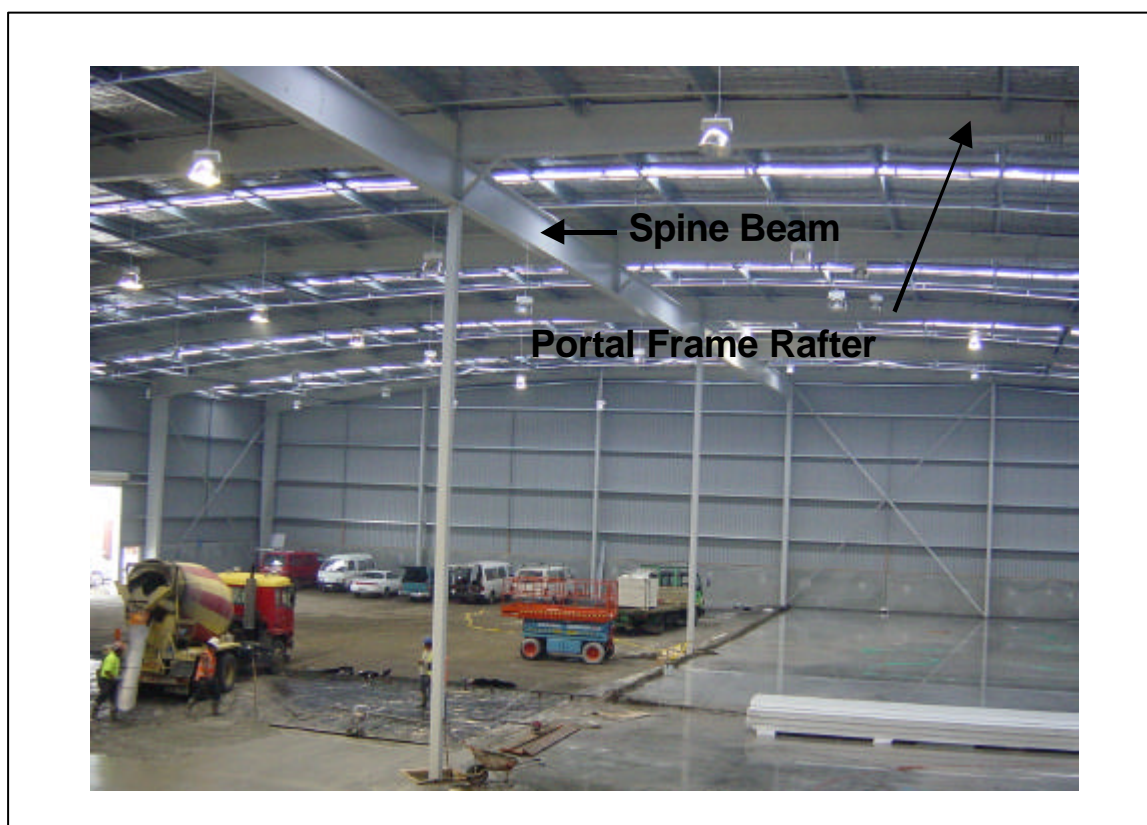
Fig. 73.3 Example of Spine Beam in Portal Frame Building
