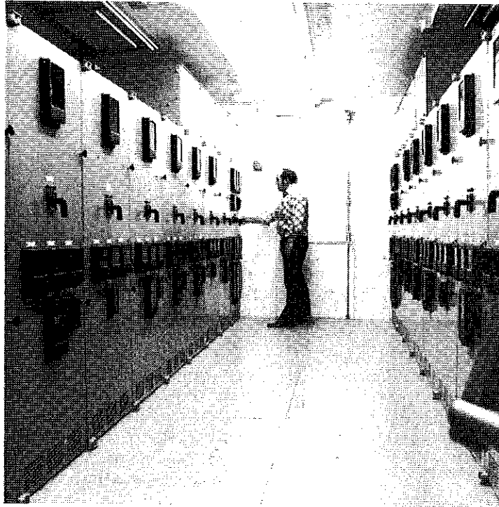
Figure 1. 5 KV Indoor Switchgear Installation
