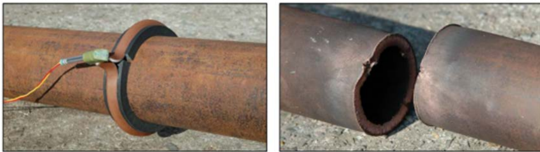
Figure 10.19 Flexible Linear Shaped Charge about Pipe Circumference, Before Detonation and After Detonation [149]
