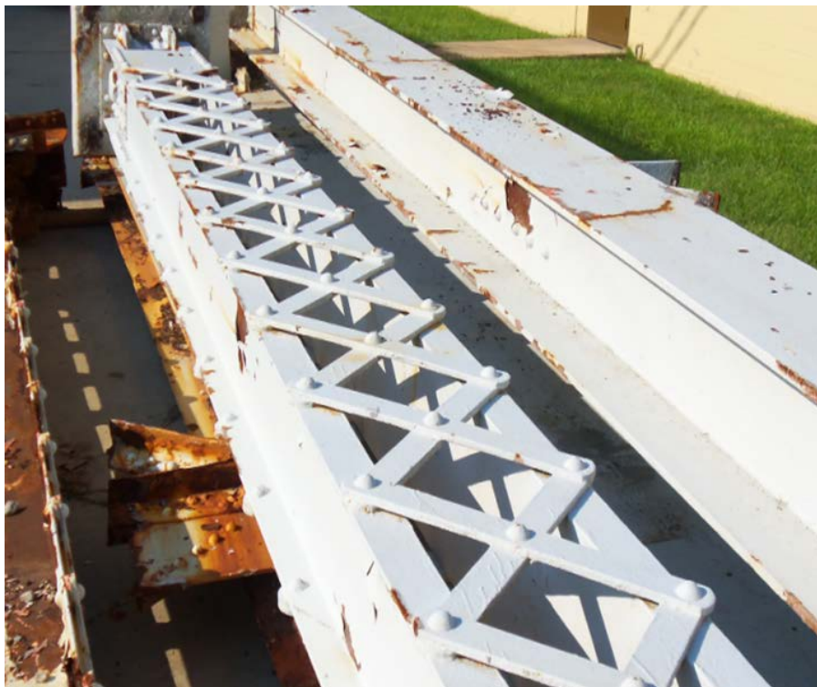
Figure 11.2 Example of Steel Laced Column [157]
