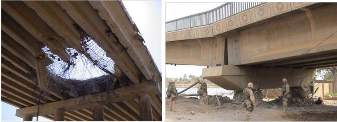
Figure 1.3 Illustration of Blast-Damaged Bridges, (left) Bridge Deck Breach Due to Above-Deck Detonation [19], (right) Catastrophic Failure of Bent Columns Due to Below-Deck Detonation [20]
