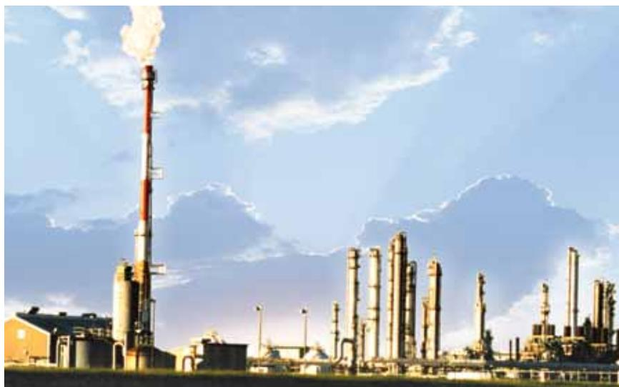
▲ **Figure 1.** Typical elevated single-point flares fire upward.
