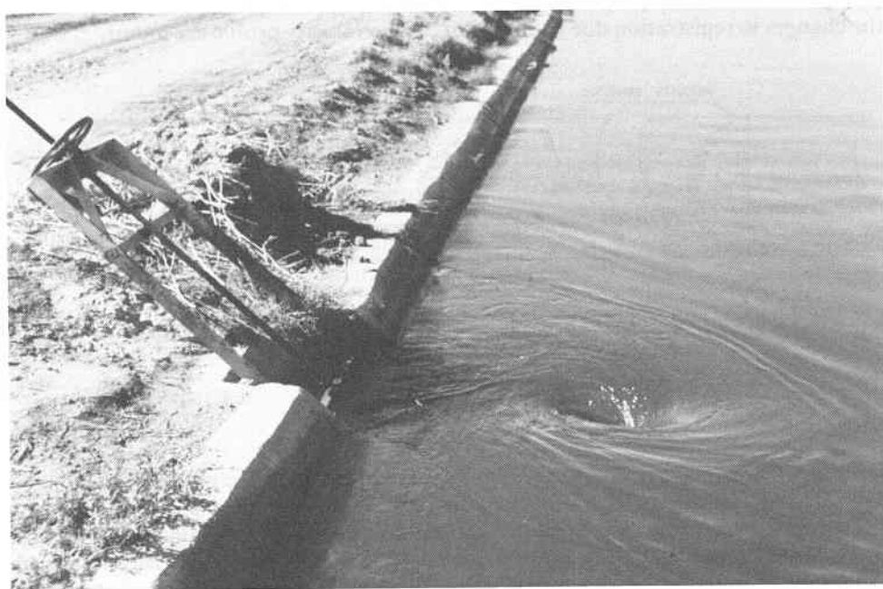
Photo 5 To avoid such a vortex the gate opening must be sufficiently deep below the upstream water level
