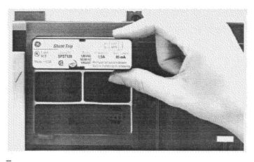
Figure 3. Inserting a Shunt Trip into the accessory compartment.
