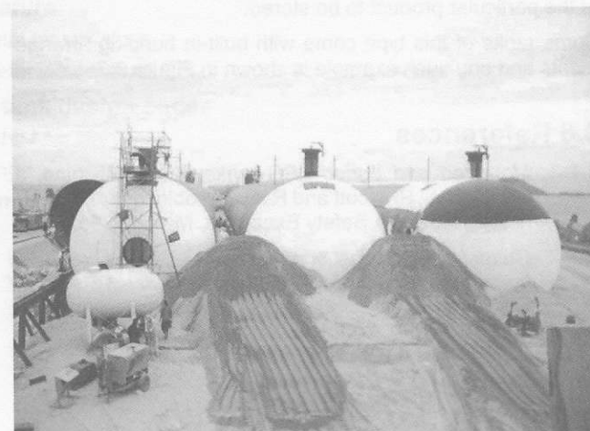
Figure 9.6 Mounded storage tank being laid on prepared sand beds Courtesy of
