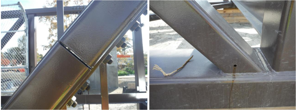
Figure 2.4.1.3-1—Example of a poorly detailed HSS pedestrian bridge: (a) splices allow moisture to enter the inside of closed sections (b) drain holes are placed too high on the vertical and diagonal members, allowing water to pond on the inside below the drain holes.
