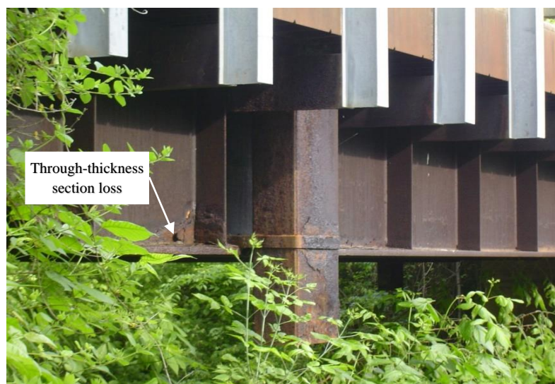
Figure 2.3.2-2—Vegetation surrounding UWS bridges increases local humidity and can trap debris, leading to section loss.
