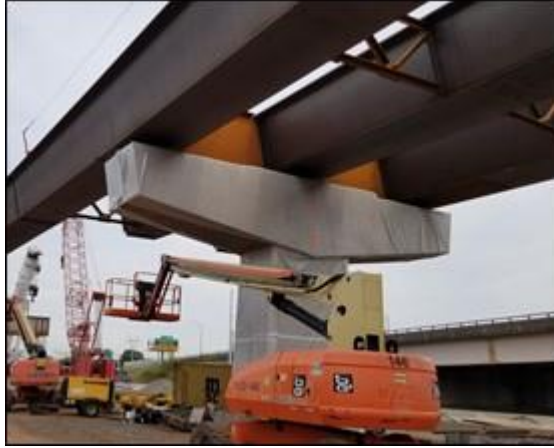
Figure 3.5.2-1—Example of wrapping a concrete pier during UWS girder construction.
