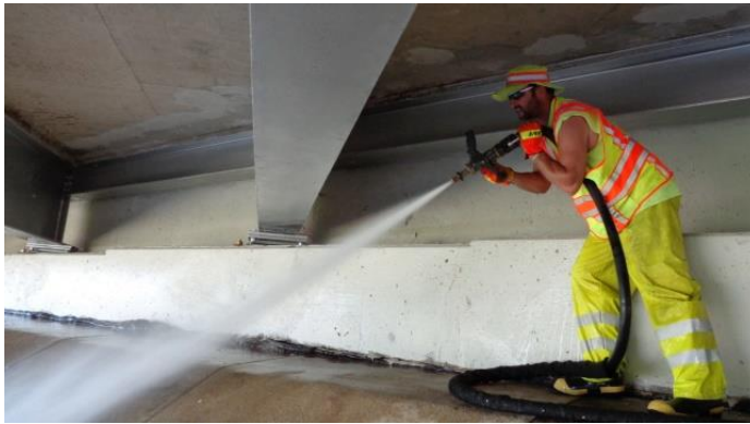
Figure 5.1.3.2.1-3—Substructure cleaning.
