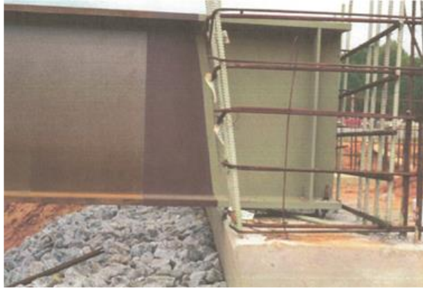
Figure 2.5.1-1—Coating protection for portions of weathering steel embedded in concrete.
