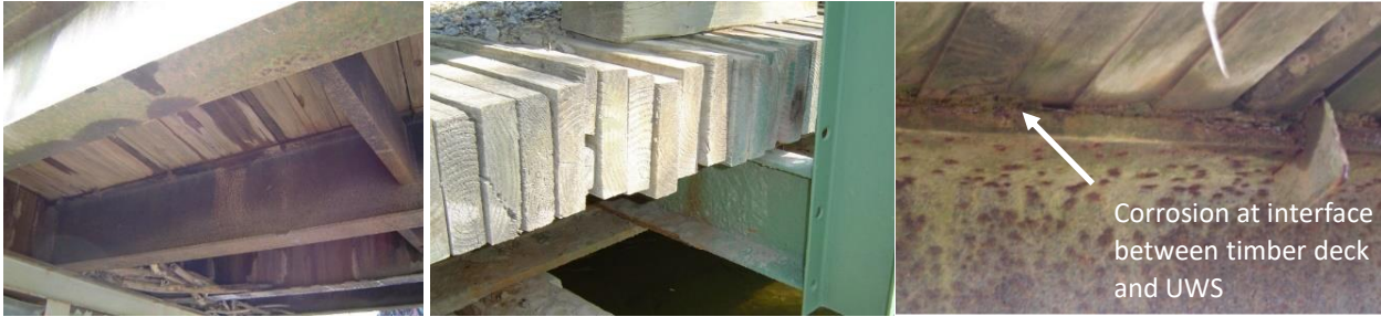
Figure 2.4.4-1—Timber decks retain moisture (as shown on the left), which can lead to blistering paint (middle) and accelerated corrosion of UWS (right).
