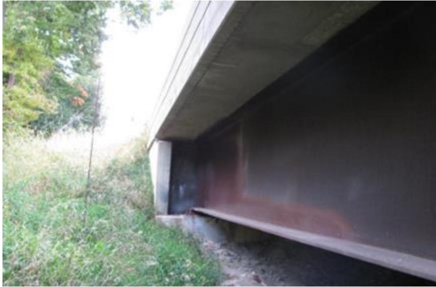
Figure 6.1.1-4—Example spot painting of UWS girder end attributed to effects of a leaking joint.
