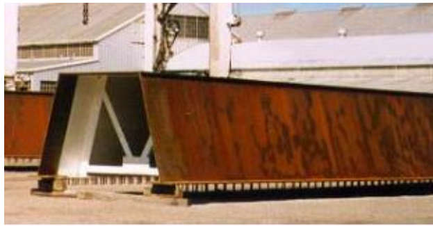
Figure 3.1.1-2—Incomplete blasting of a bent cap.
