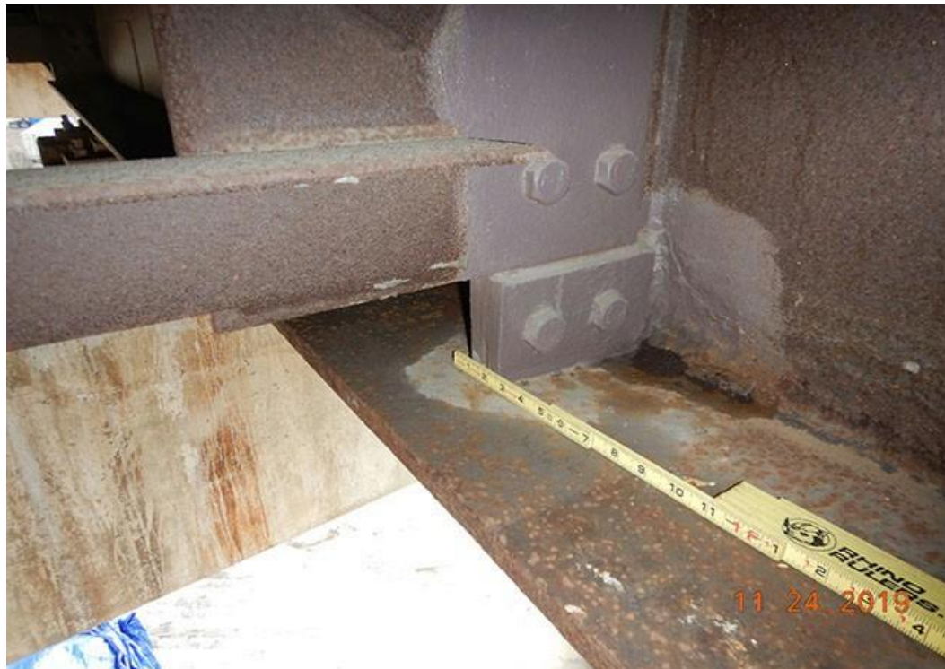
Figure 6.1.1-3—Painted weathering steel around a connection plate without drain clips.
