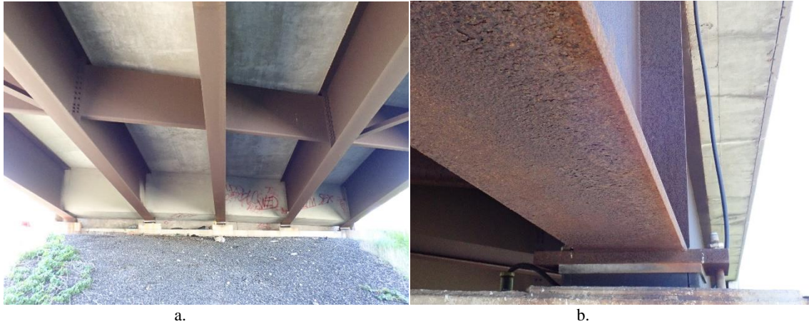
Figure 4.1.1.2-1—Sight distance is critical for an accurate determination of UWS performance. A view from ground level approximately 20 ft. in (a) could lead to a markedly different conclusion than the same structure inspected from a closer distance (b).
