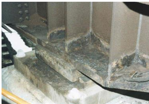
Figure 2.5.1-4—(a) Debris and moisture traps formed by bearing stiffeners without drain holes; (b) stiffeners fabricated with clips to reduce debris and moisture accumulation.
