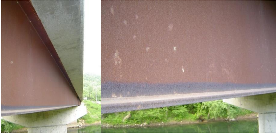
Figure 2.4.5-1—Relatively narrow deck overhangs (left) can cause ponded water on bottom flanges, which is drawn up the web by capillary action, and accelerates corrosion (right).
