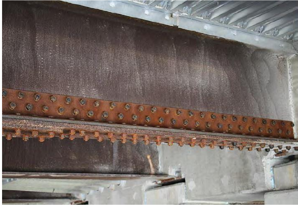
Figure 6.1.3-1—Bolted angle repair to strengthen a UWS beam bottom flange.
