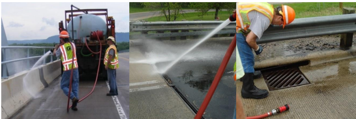
Figure 5.1.3.2.1-1—Deck component cleaning (a) roadway and parapet (b) expansion joint (c) drainage components.
