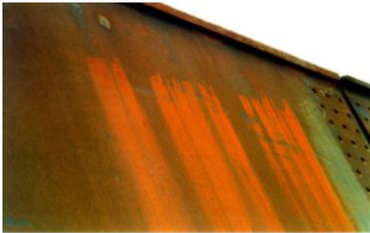
Figure 3.1.1-3—Non-uniform appearance caused by spot re-blasting.
