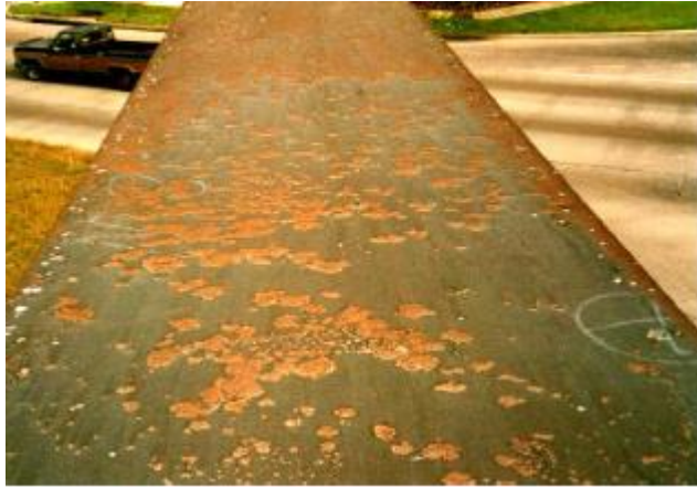
Figure 3.1.1-2—Incomplete blasting of a bent cap.
