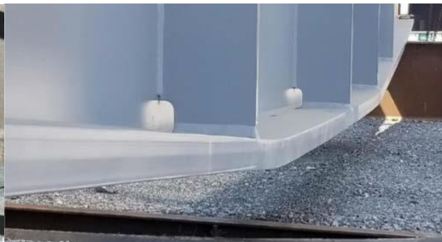
Figure 2.5.1-4—(a) Debris and moisture traps formed by bearing stiffeners without drain holes; (b) stiffeners fabricated with clips to reduce debris and moisture accumulation.
