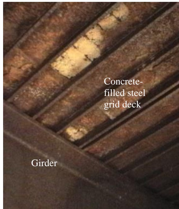
Figure 2.4.4-2—Concrete filled steel grid deck, without overfill, viewed from bottom, shows that bottom plate of deck has broken loose from water infiltrating between steel grid and concrete fill.
