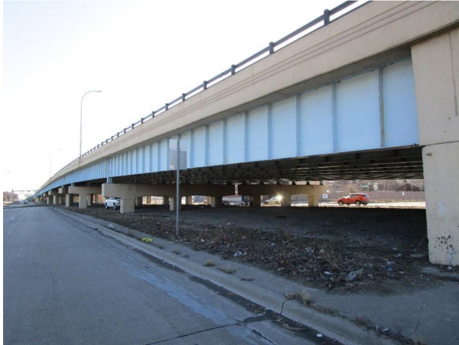
Figure 6.1.1-5—Weathering steel bridge with entire superstructure painted.
