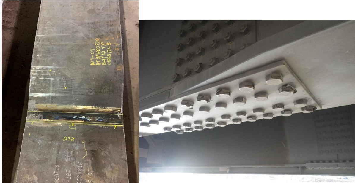
Figure 2.4.7-1—Flange width transitions often result in the optimized design from a strength perspective, particularly for curved bridges.
