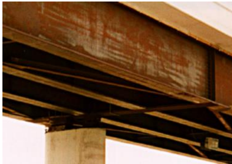
Figure 3.1.1-1—Non-uniform mill scale removal.
