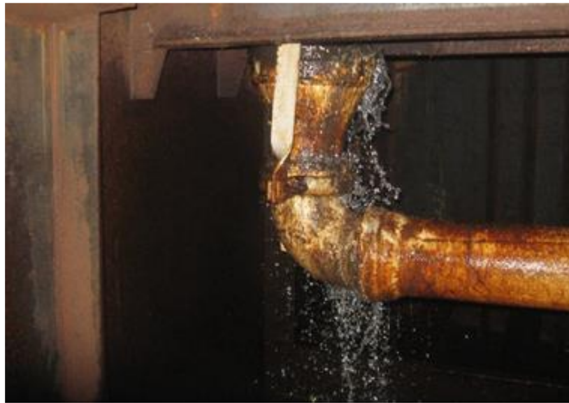
Figure 2.5.1-9—Clogged and leaking drain.
