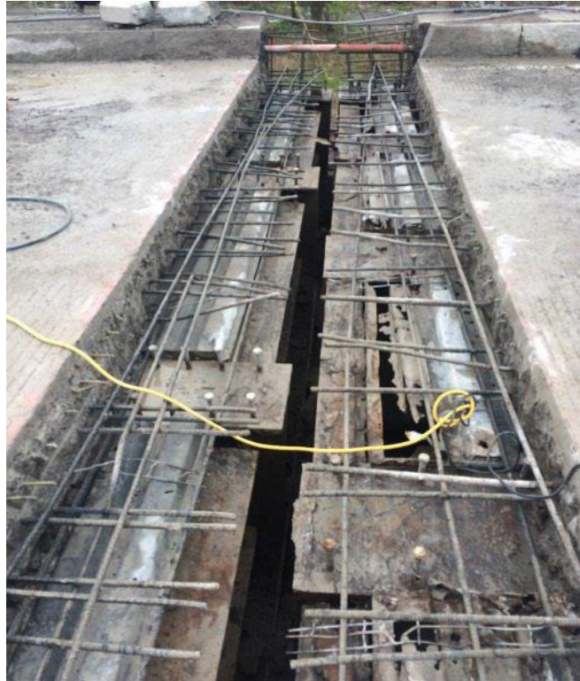
Figure 6.1.4-1—Link slab construction on existing bridge.
