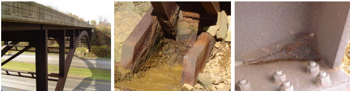
Figure 2.4.1.4-1—The drainage path of inclined members needs consideration. The middle and right photos show the consequences of water ponding at the termination of inclined members where no drainage was provided.
