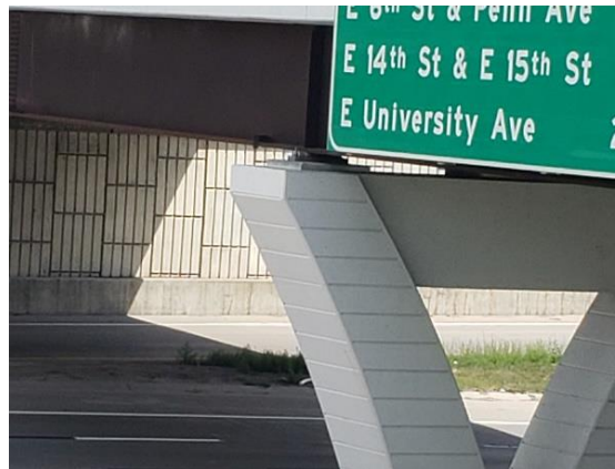
Figure 3.5.2-2—Example of a concrete pier that was wrapped during construction and sealed post-construction. The bridge is approximately 20 years old at the time of the photo.
