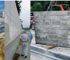
Sound and impact panels along railroads/highways in US
