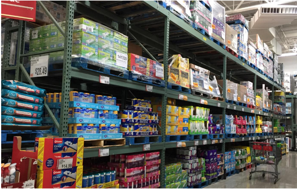
Figure 1: An industrial rack structure with perforated cold-formed steel columns
