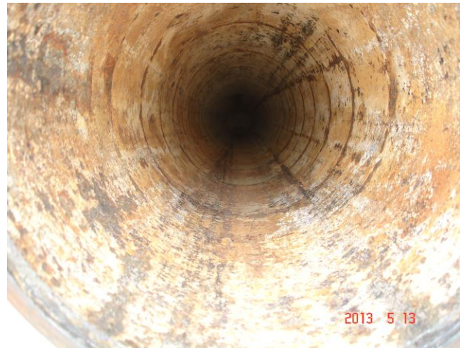
The shell internal surface was dirty and corroded
