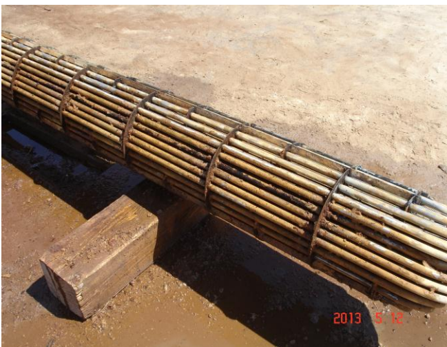
The tube bundle during cleaning
